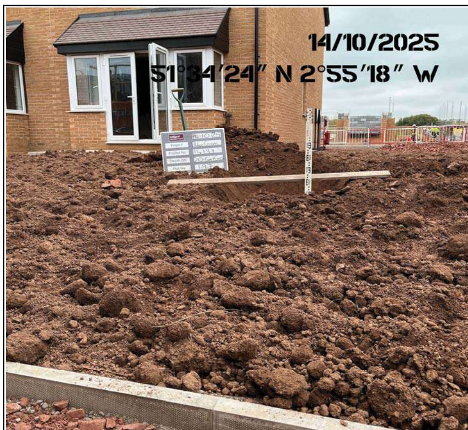
Plot 197 Soil capping Depth Check
