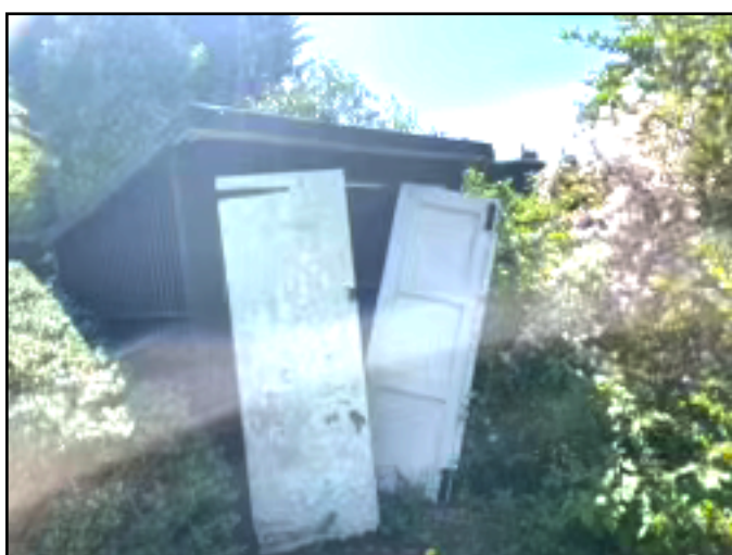
Figure 3.1. View of Storage Shed
