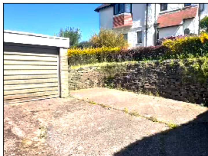
Photo 11. Garage and hardstanding area. View from roadside along south of site.
