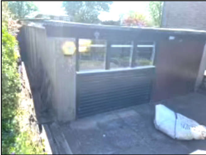
Figure 3.3. View of Rear Elevation of Garage
