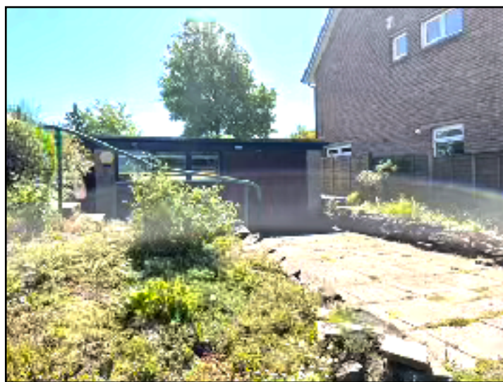
Photo 10. Rear view of garage structure and patio area in west of site.
