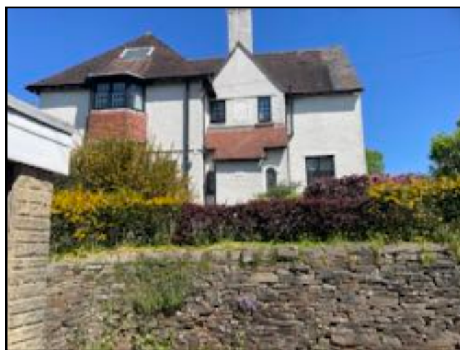
Figure 3.2. View of Main House
