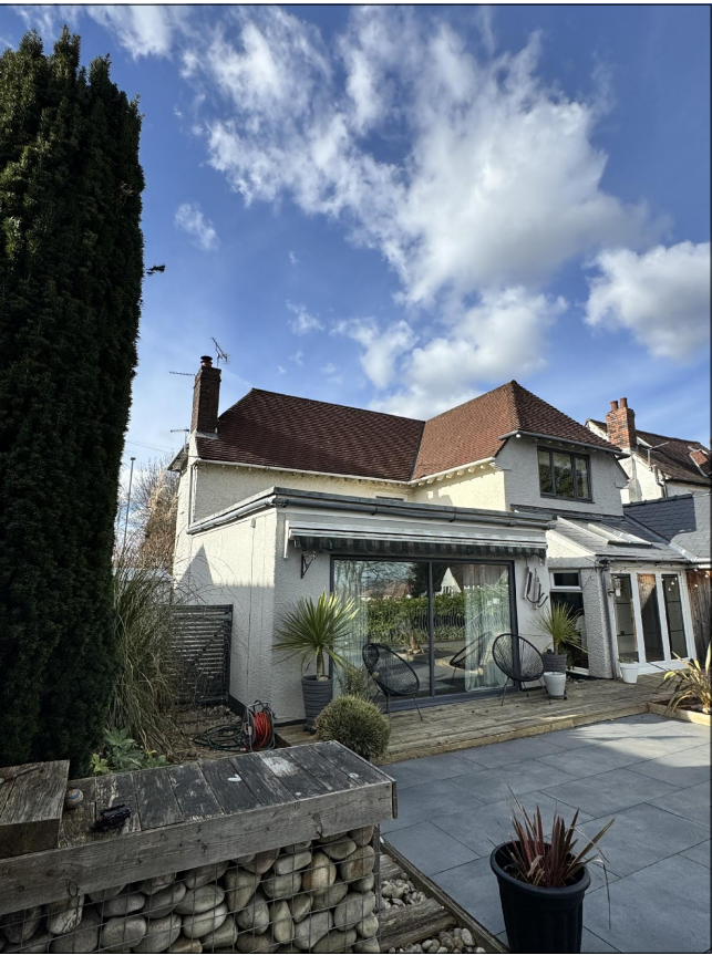
Image for the existing flat roof to be removed.
