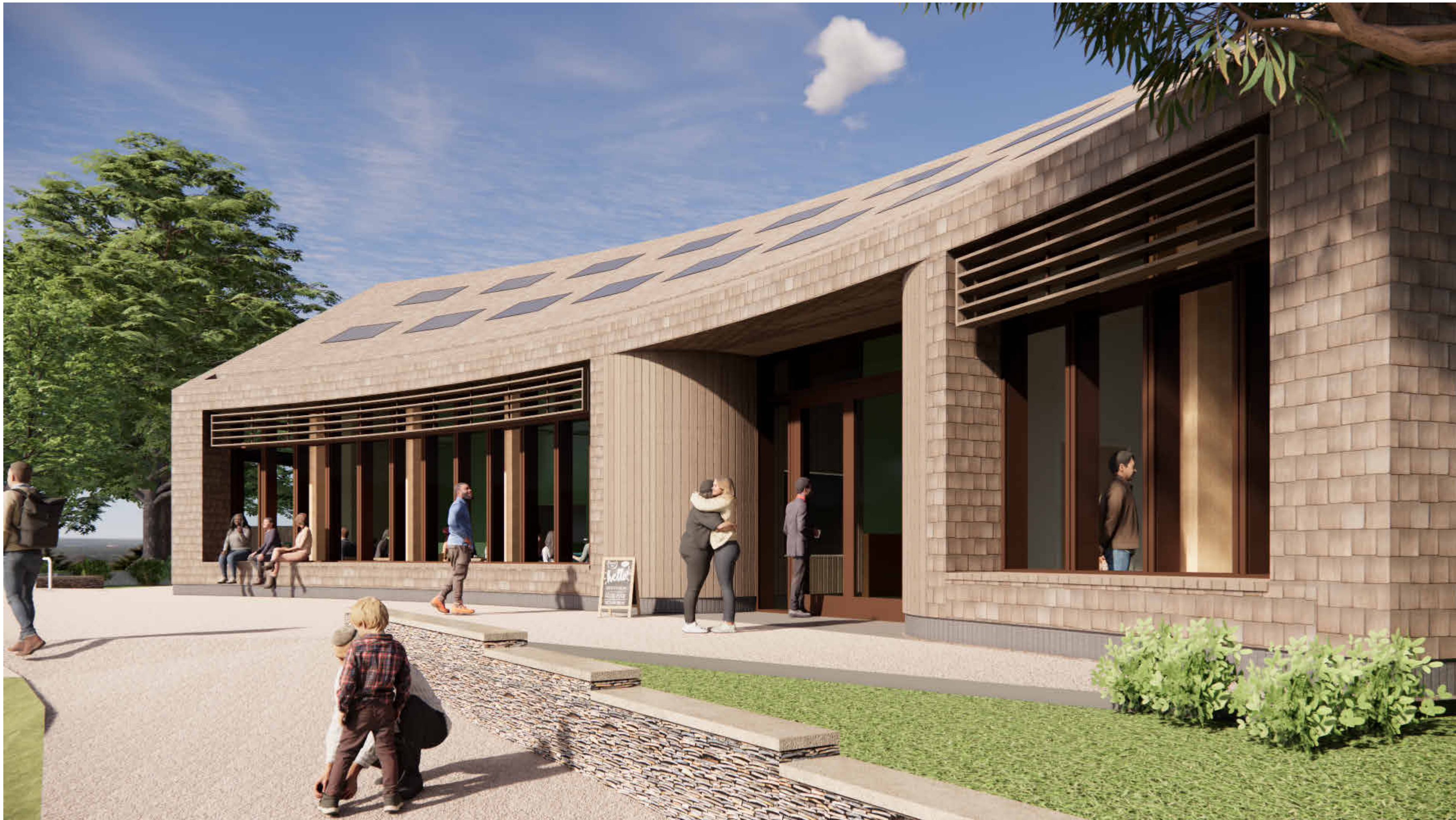
View towards West of Site
