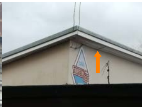
Gap into soffit
