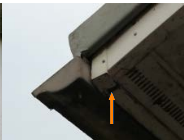
Gap into soffit
