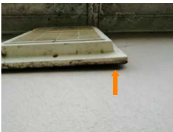
Gap between shutter and barge board
