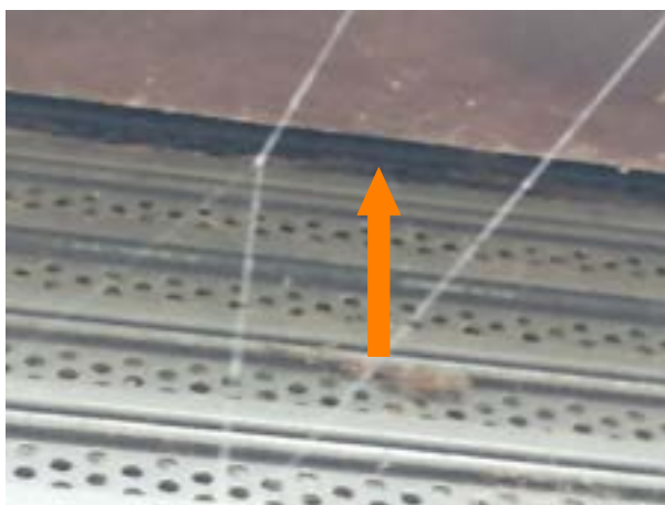
Gap between shutter and barge board
