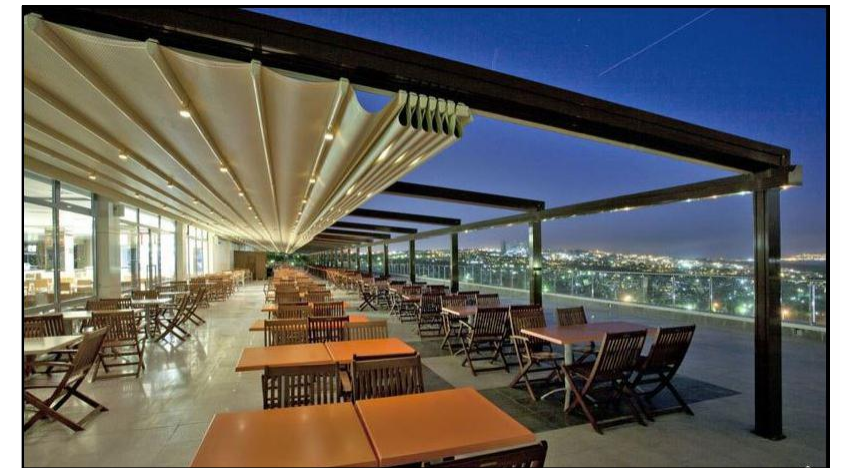
RETRACTABLE TENSILE STRUCTURE
