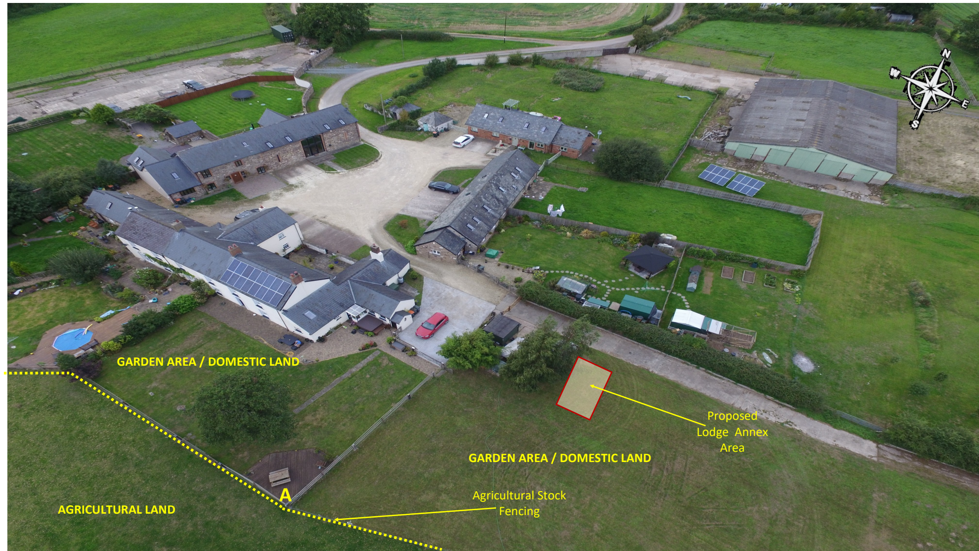
Image Showing Land Usage Separation Boundary As Historically Defined (Photo 2017)
