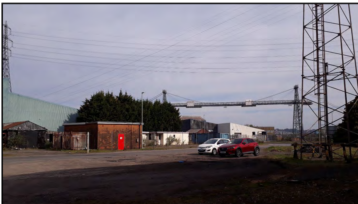
Plate B. View to north showing the existing brick substation (left of centre), the Transporter Bridge and pylon lines, lighting column (right) and trees along the northeast boundary
