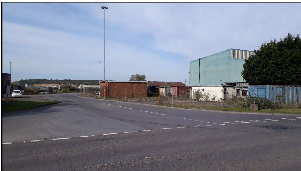
Plate C. View to north-northwest showing with the existing brick substation, structures and container units, The T-junction of E Way Road with Alexandra Dock Road and the north warehouse
