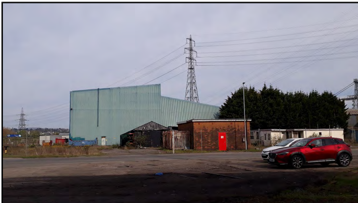
Plate A. View to northwest showing the existing brick substation (right of centre) and other site buildings with the north warehouse behind
