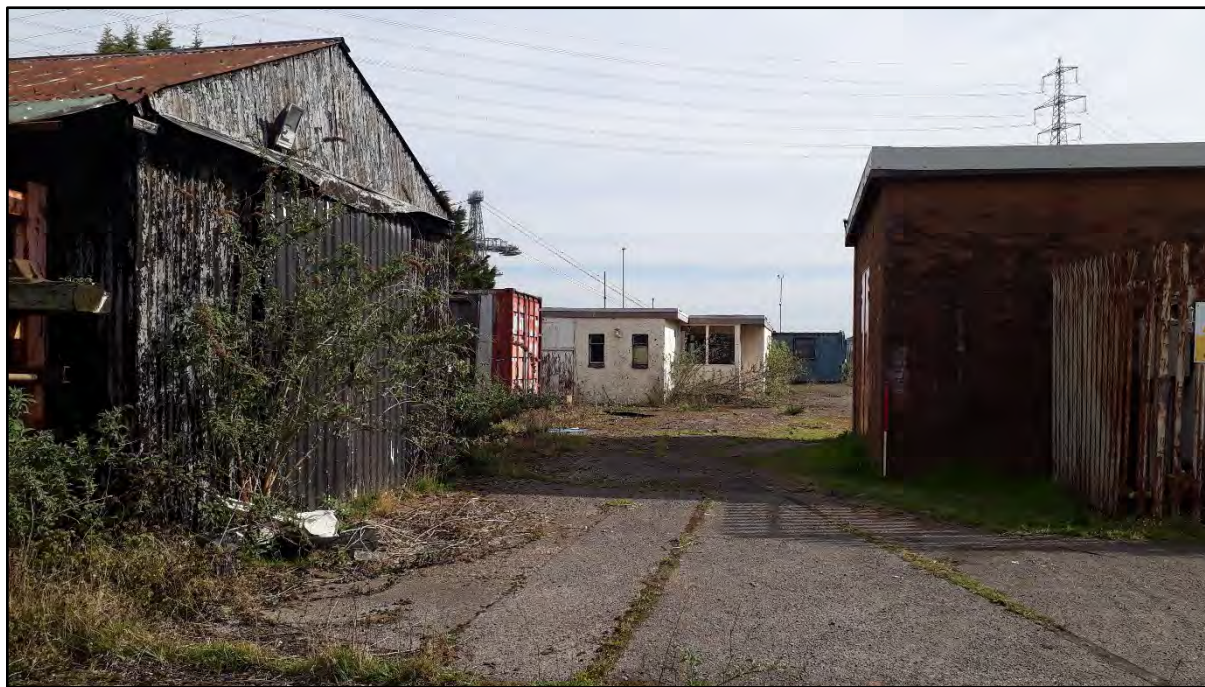
Plate G. View to northeast between the existing brick substation (right), shack (left) and demountable office building (centre rear)
