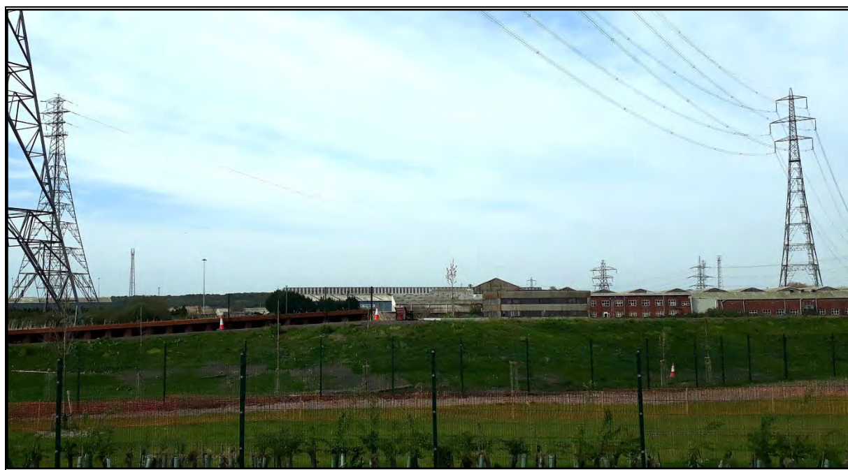
Plate H. View to northwest from Coronation Park toward the site. The site is behind the left traffic cone where one of the lighting columns in the scrub can be seen.
