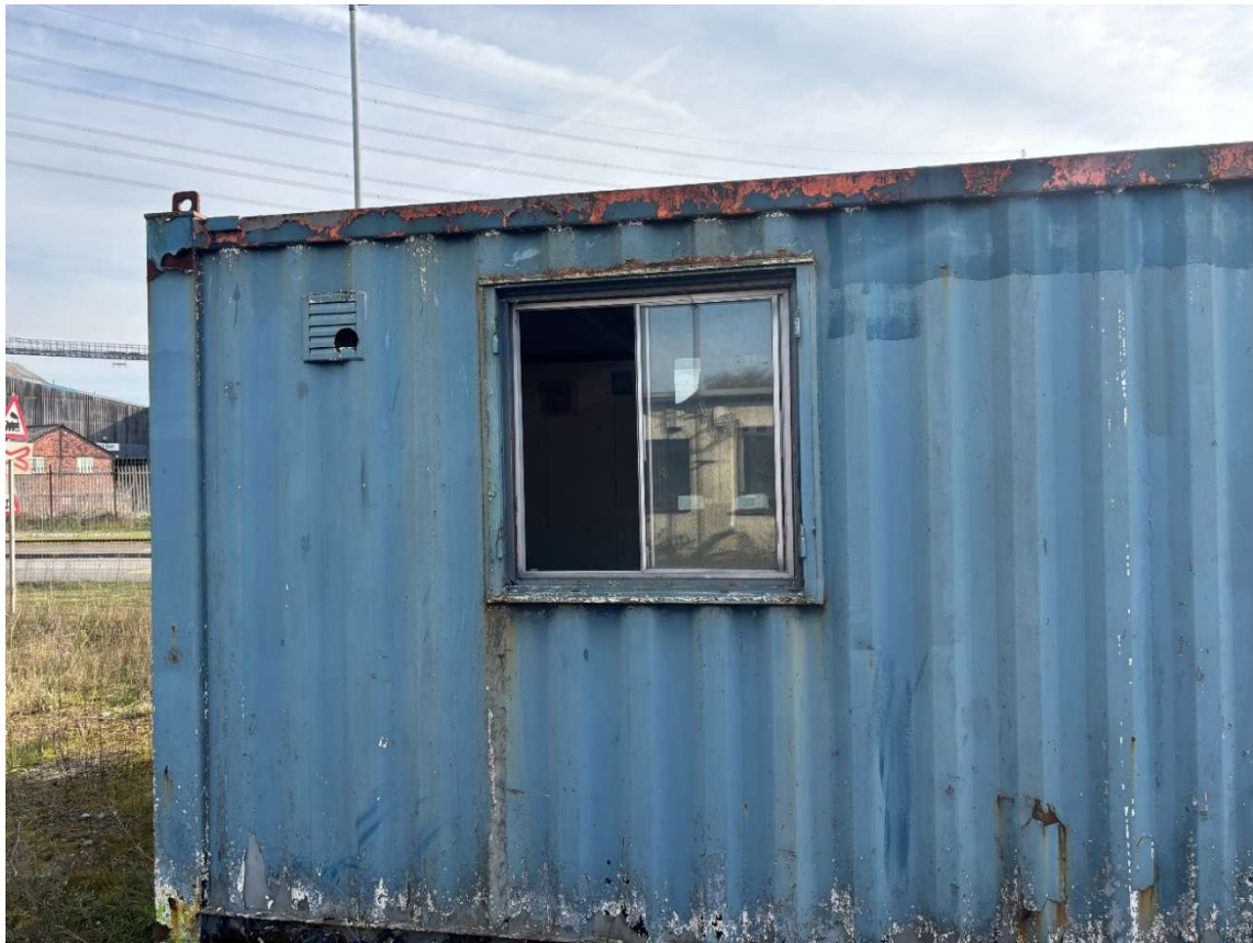
6.3.9 Image 9 - Corrugated office container showing open window (Target Note 5)
