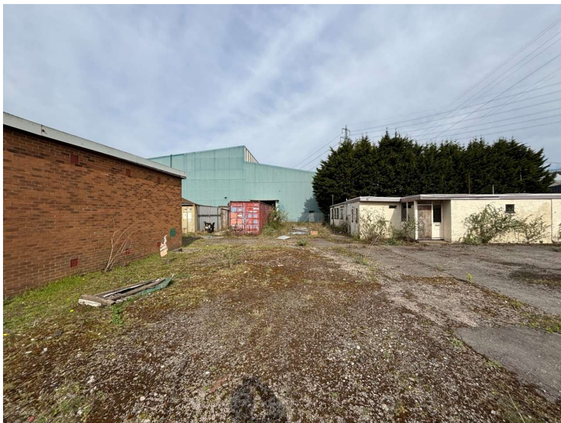
Image 2 - Central view of substation and cabin office
