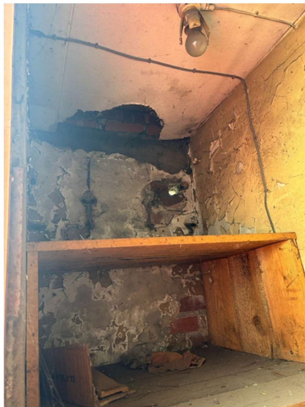
Image 6 - Entrance to loft space in office cabin (Target Note 1)
