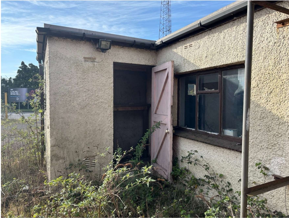
Image 5 - Office cabin with open door (Target Note 1)
