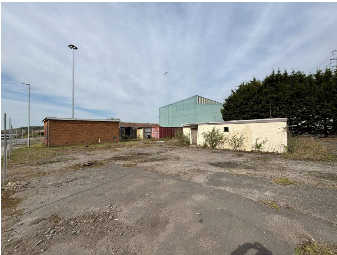
Image 1 - View of substation and office cabin
