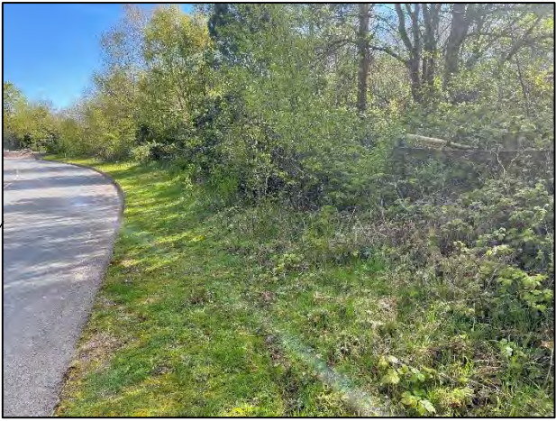
Mature and impenetrable vegetation is present in front of the fence line along the majority of this section, with evidence of public access restricted to areas where vegetation is less dense. Gaps in existing perimeter fence to be infilled and fencing upgraded (where appropriate) where public access has been noted, avoiding impacts to vegetation as far as practicable.
