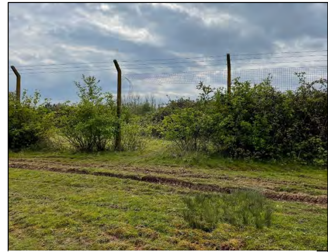
Existing fence line to be repaired (like-for-like) where gaps have been cut/opened up to restrict future access (example in photo above).
