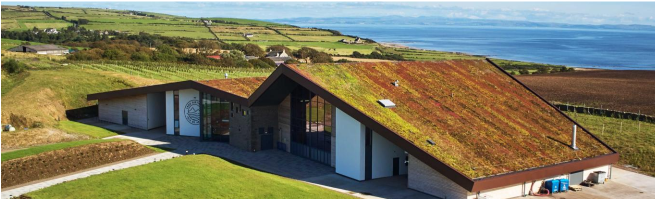
Figure 1: Example of the Bauder Extensive Lightweight Sedum XF 301 roof implemented in Scotland.
