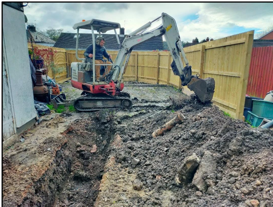
Figure 8: Excavation of Trench 1, facing south-east.
