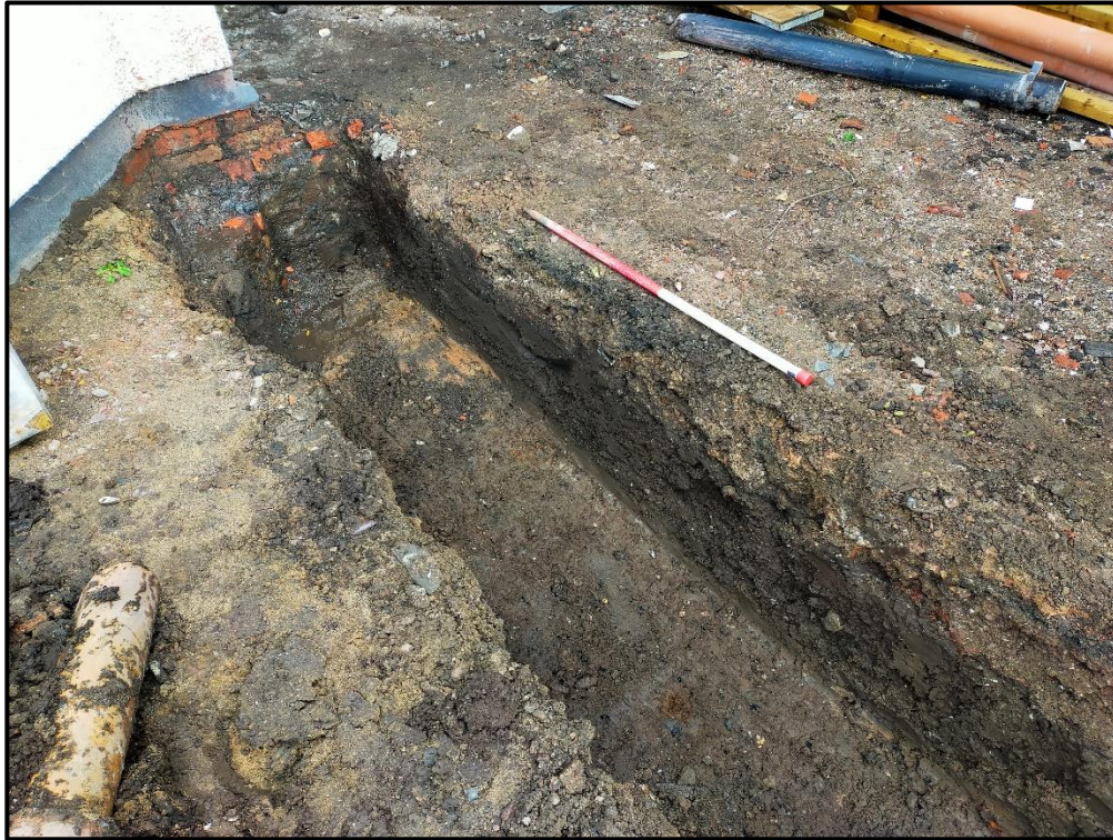
Figure 10: Brick foundations for house [104], facing north
