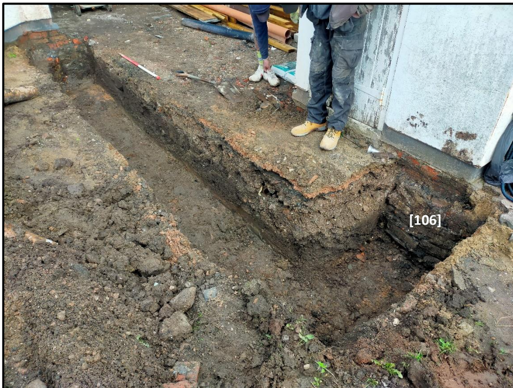
Figure 11: Stone foundations [106] beneath brick outbuilding [105] in north-eastern corner, facing north
