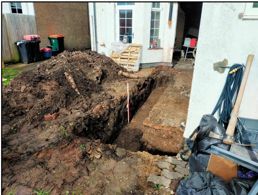
Figure 13: Trench 1 post excavation, with house beyond, facing north-west
