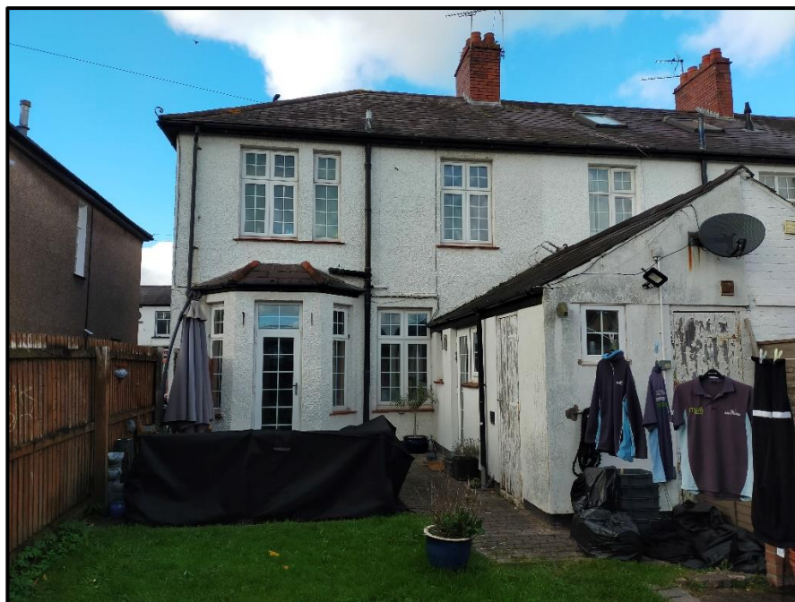
Figure 2: View of the site and rear elevation of Kia-Ora, facing north-west.
