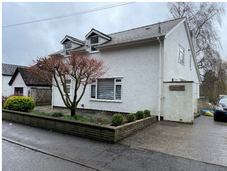
Figure 1 – Front of the property
