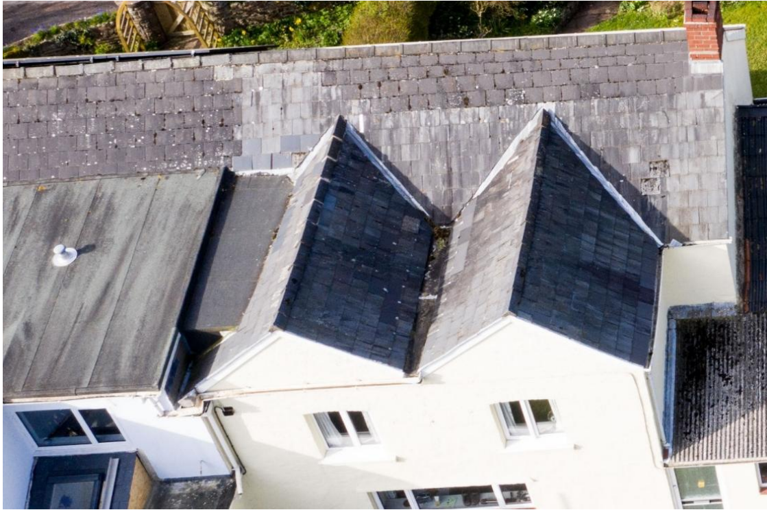
Figure 18 - Existing Roof Junction
