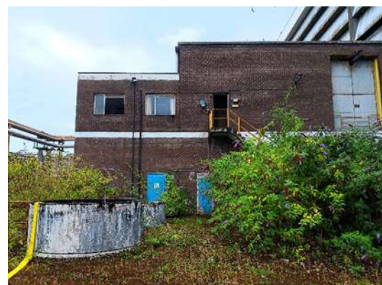
Photo 12: One of the buildings (reheat office) identified as a bat roost (on north side)
