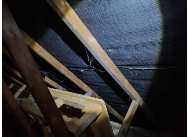
Photo 12: Lining within roof void 1 (main house) appears well sealed, with no light ingress
