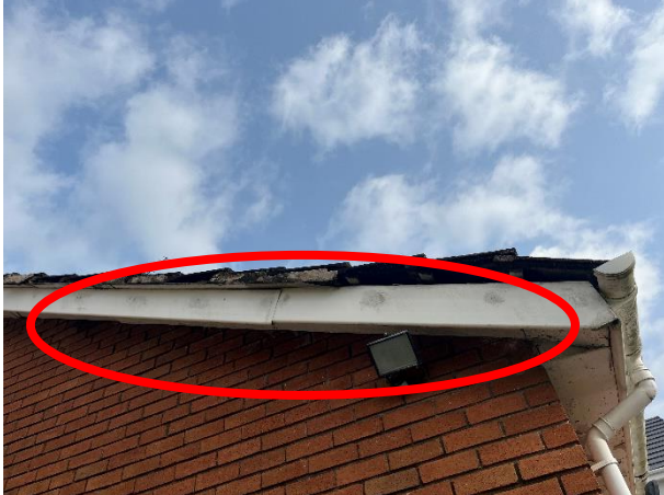
Photo 9: Roof tiles, flashing and soffit box appear well sealed on porch at southern elevation
