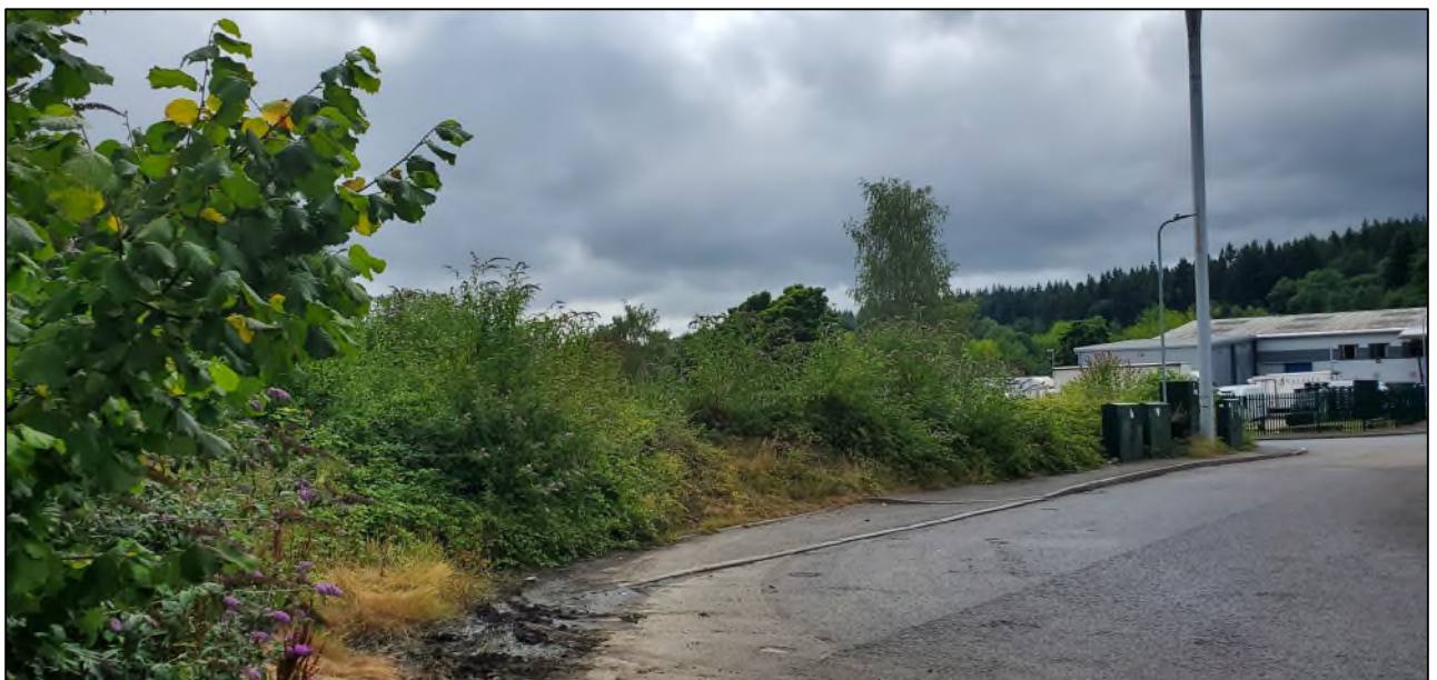
Figure 3: Silt build-up indicative of poor drainage at northern site entrance.
