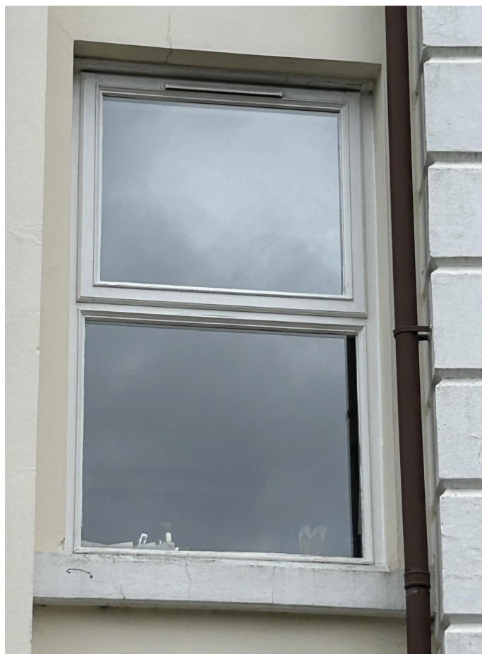
WINDOW No. W1
