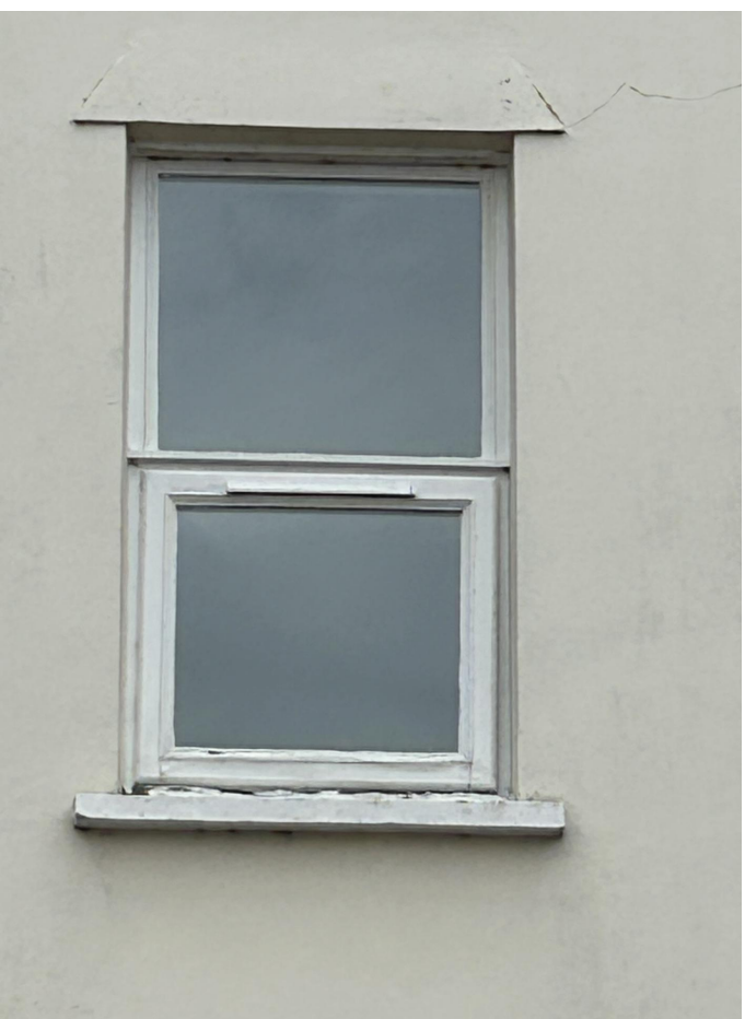
WINDOW No. W2
