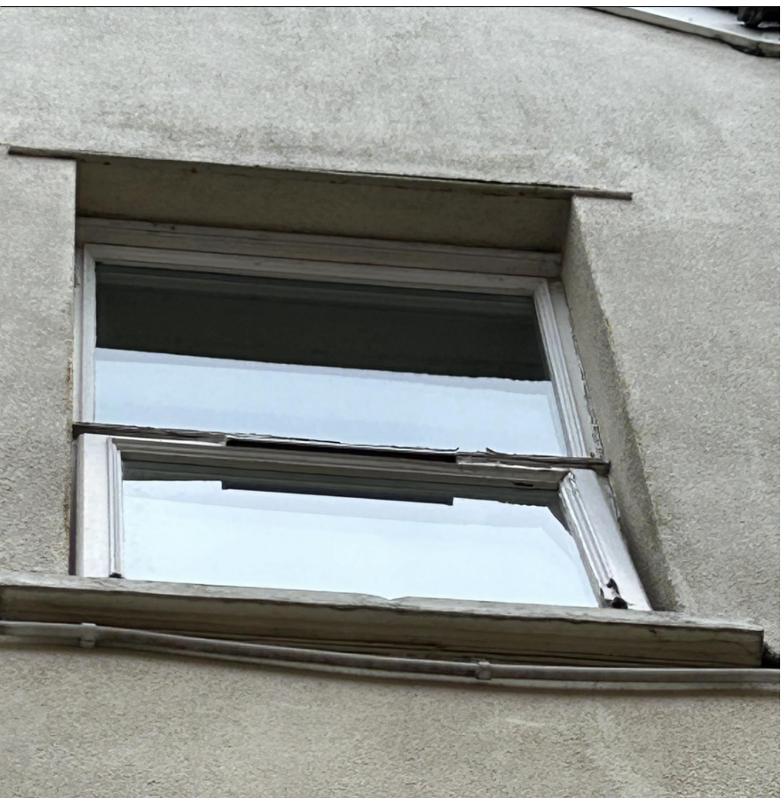
WINDOW No. W6
