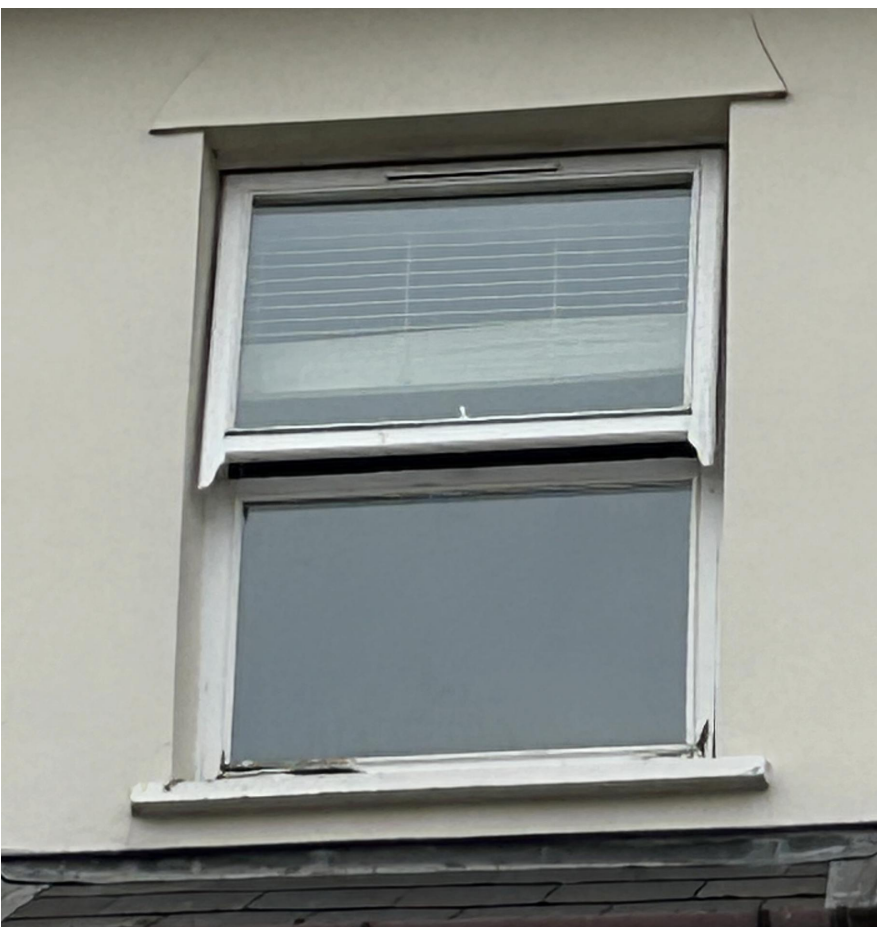
WINDOW No. W7
