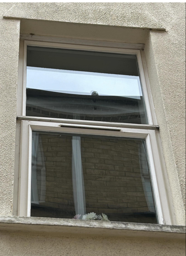
WINDOW No. W5
