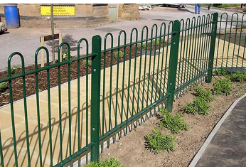
Fence to front of site
