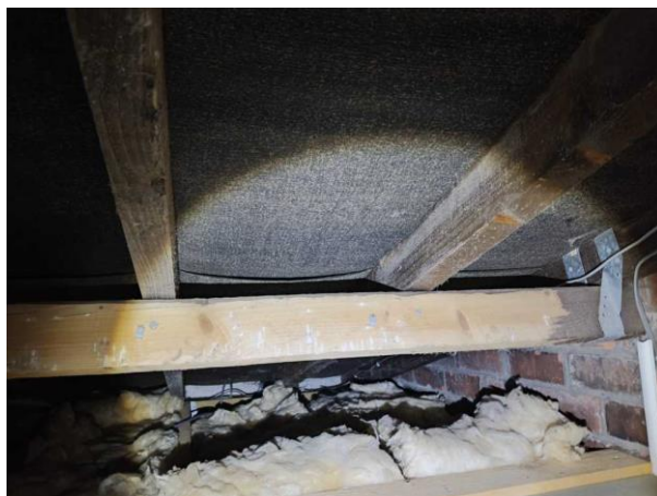
Photo 8: Internal View Of Roof And Insulation
