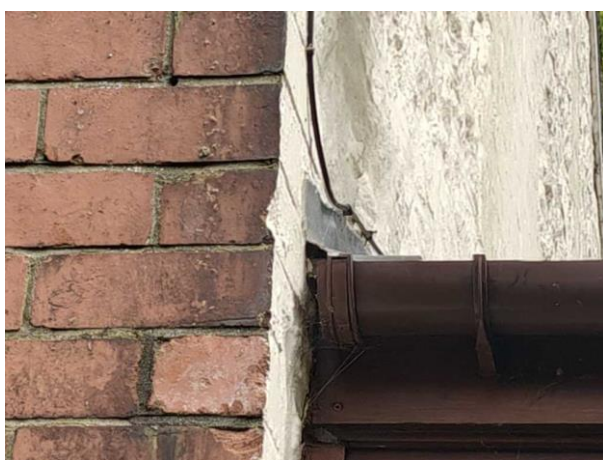
Photo 9: Lead Flashing on Southern Elevation
