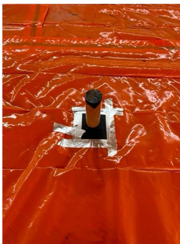
Photo 6: Example top hat/ sealed protrusions (double sided tape visible along joint (right hand photo))
