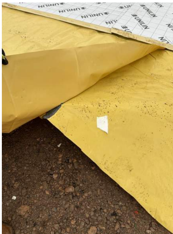
Photo 1: Section of installed membrane, insulation board and reinforcement.
