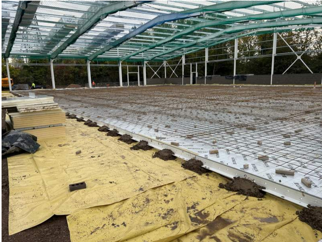
Photo 3: Subgrade in foreground with membrane, insulation, anchor joint and reinforcement shown as installed.
