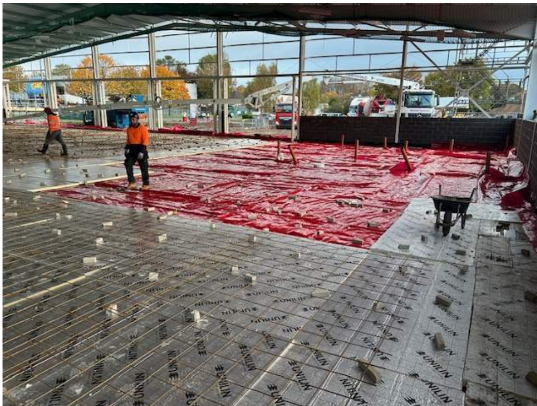
Photo 5: Final membrane area of installation. Insulation in foreground. Protrusions visible.
