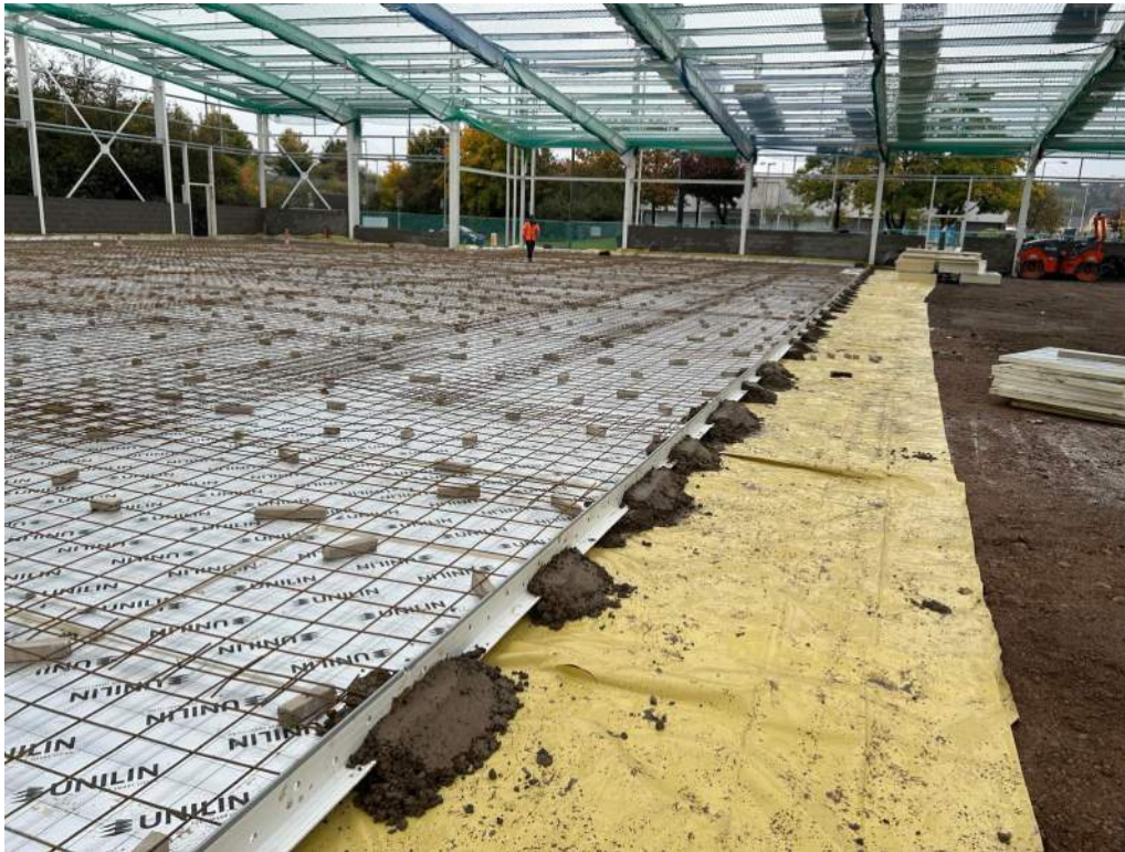
Photo 1: Section of installed membrane, insulation board and reinforcement.
