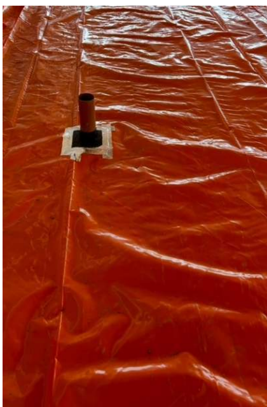
Photo 6: Example top hat/ sealed protrusions (double sided tape visible along joint (right hand photo))
