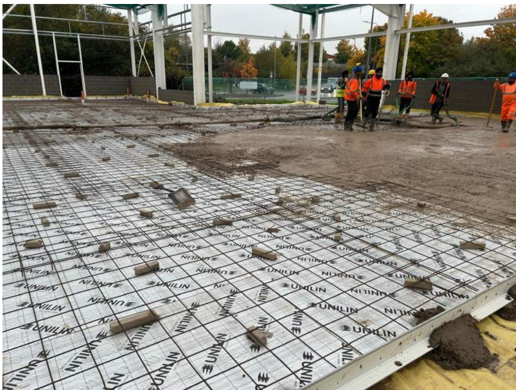
Photo 4: Pouring of concrete
