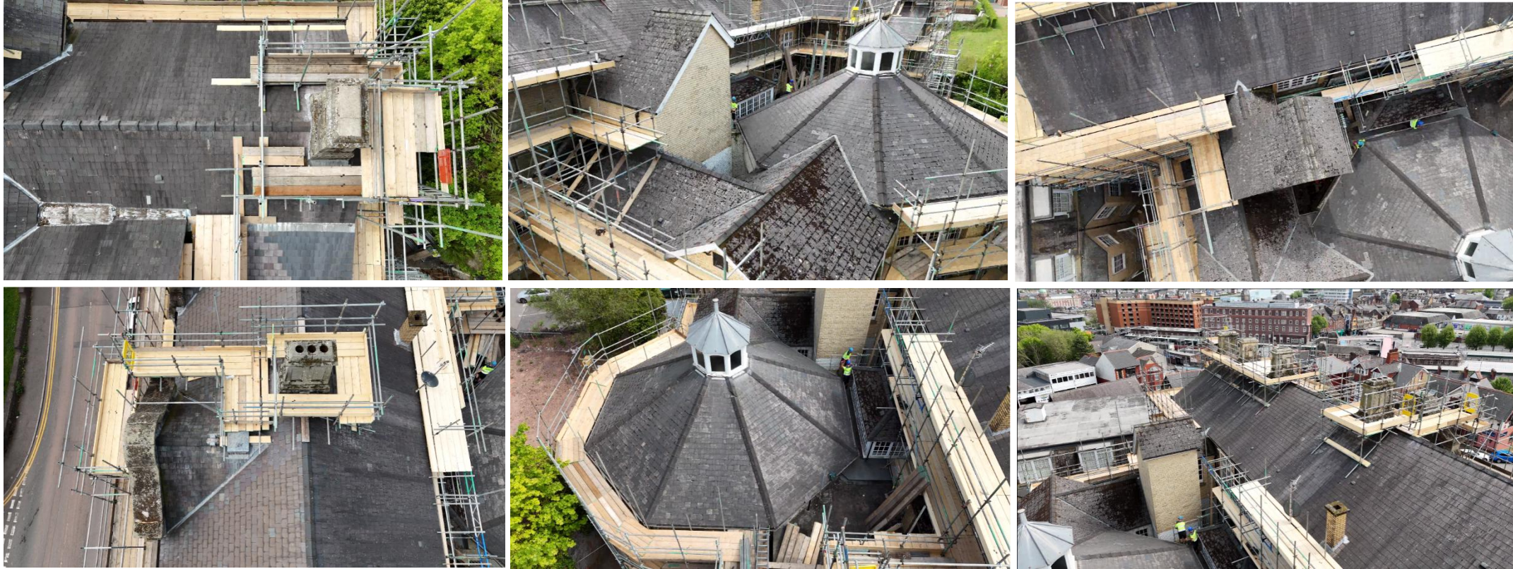
Plates 10-15: Drone survey of the roof completed
