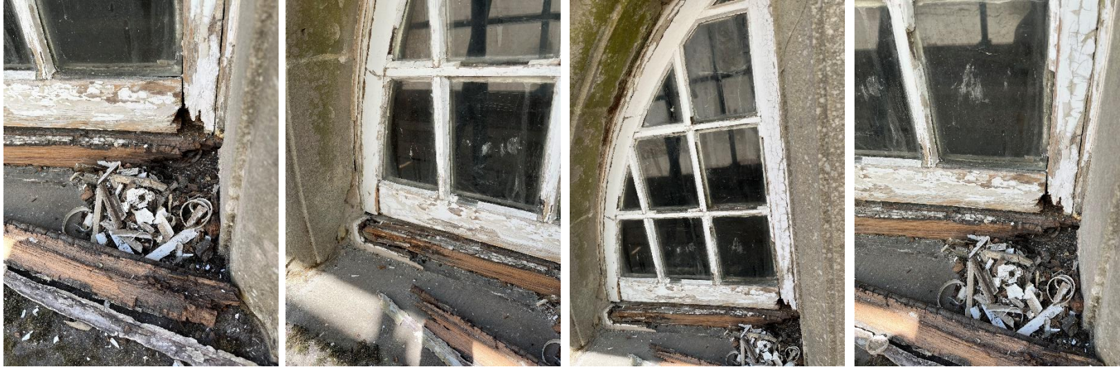
Plates 43-46: Survey of exterior joinery carried out, work started cutting out by hand rotted joinery to third floor windows
