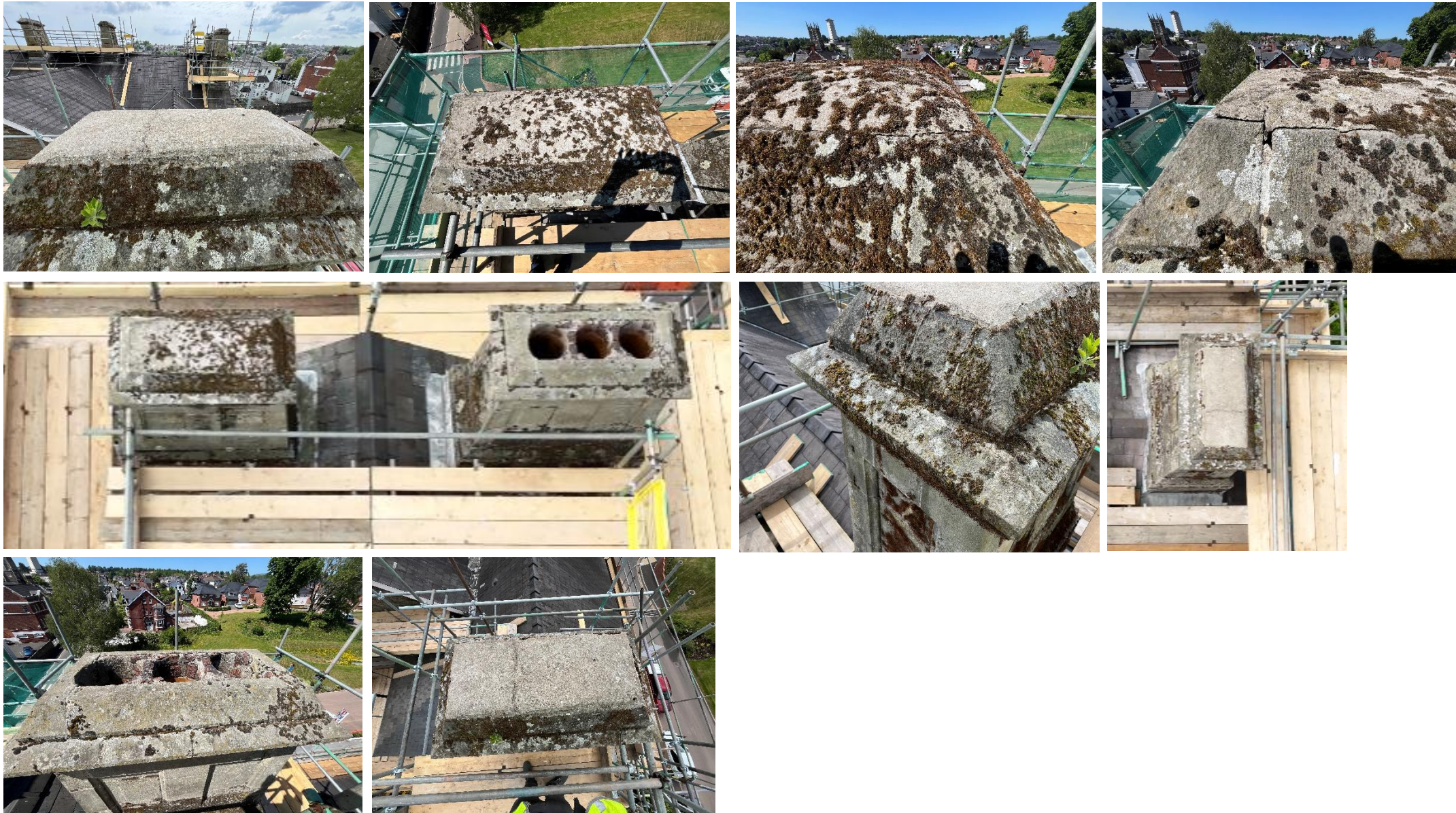
Plates 1-9: Survey of chimney cappings carried out
