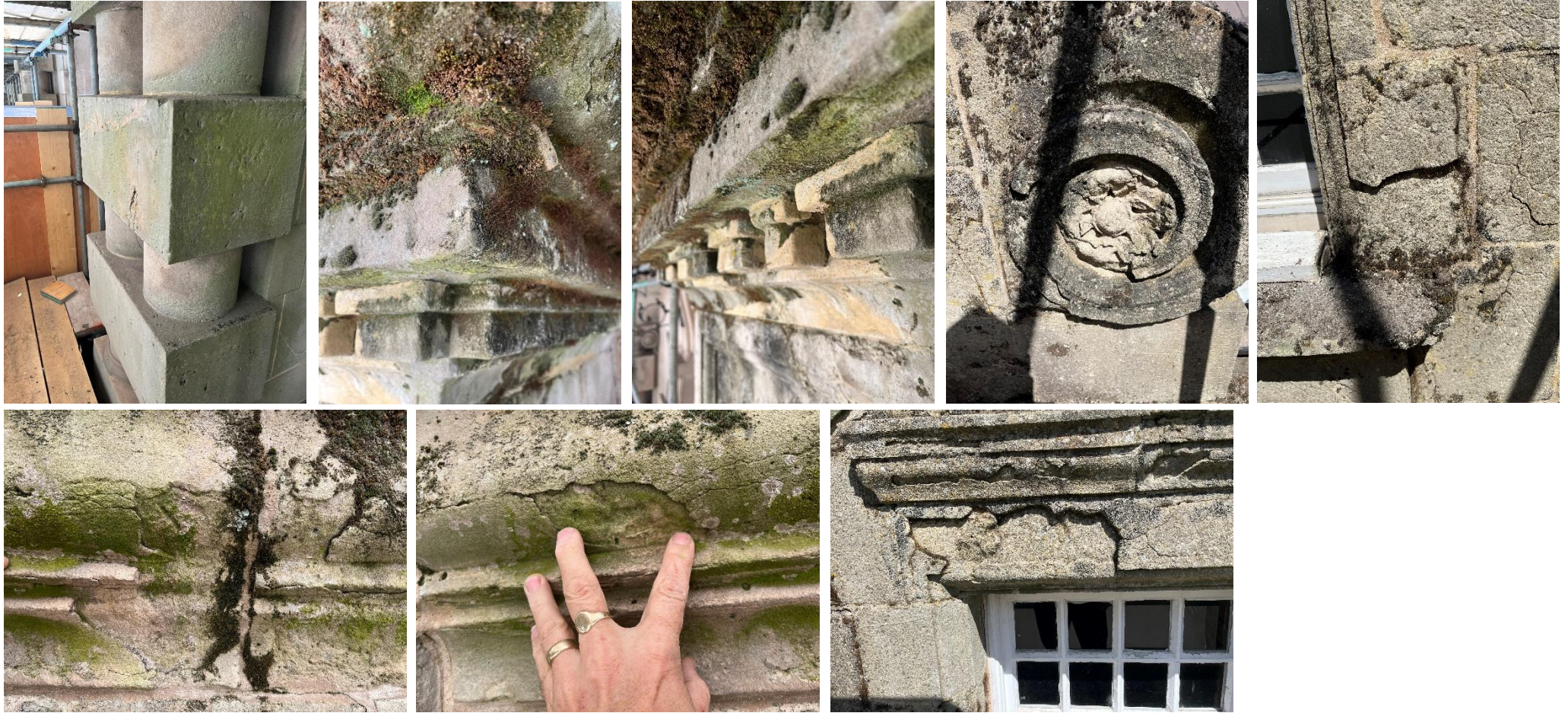
Plates 25-32: Survey of exterior stone works carried out
