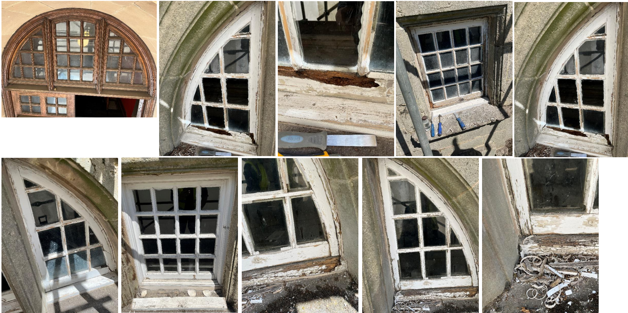
Plates 33-42: Survey of exterior joinery carried out, work started cutting out by hand rotted joinery to third floor windows
