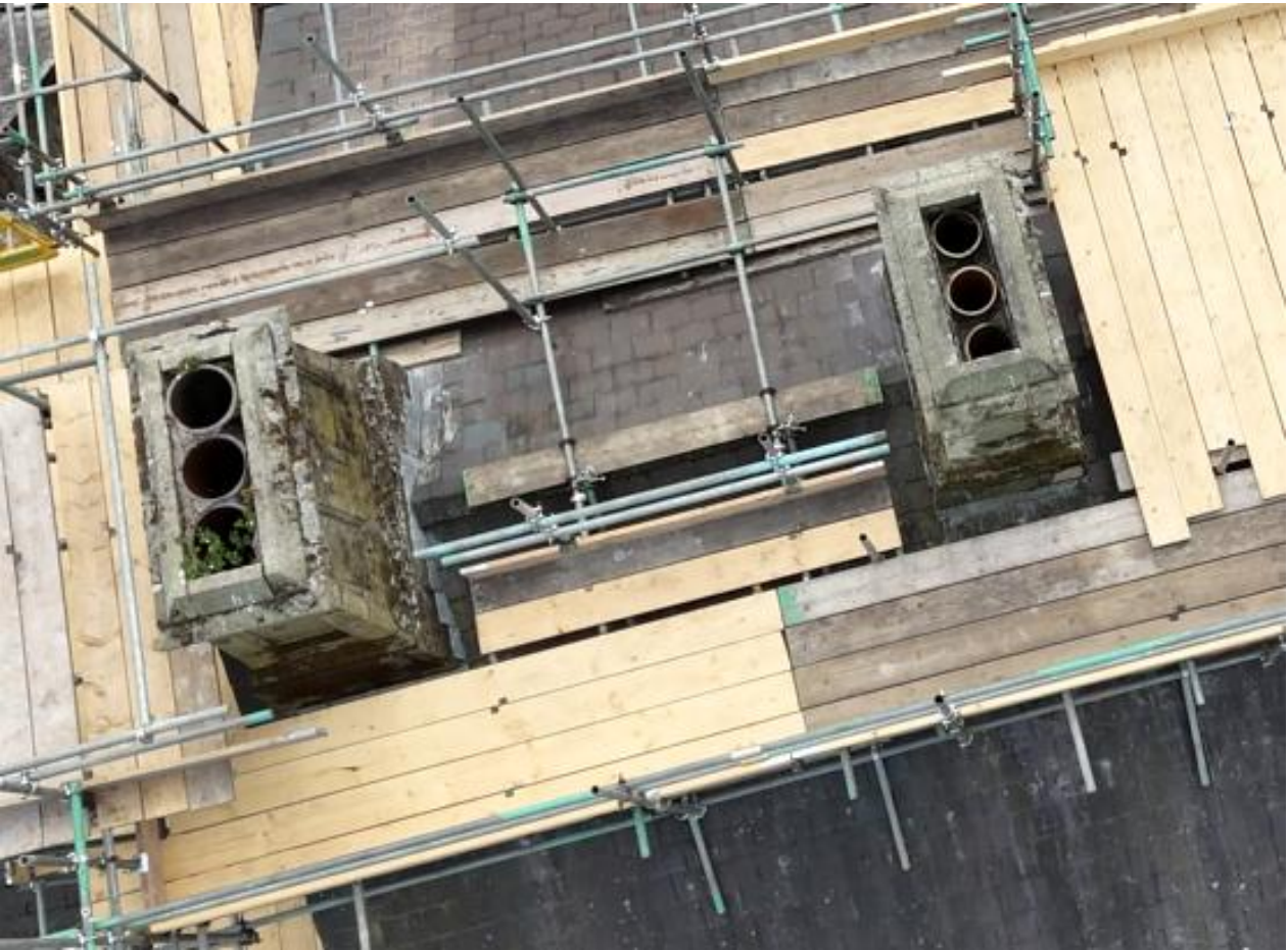
Plate 5: Uncapped stacks viewed from drone footage, estimated border stone toppers of 50mm from pylonic sloped side.
