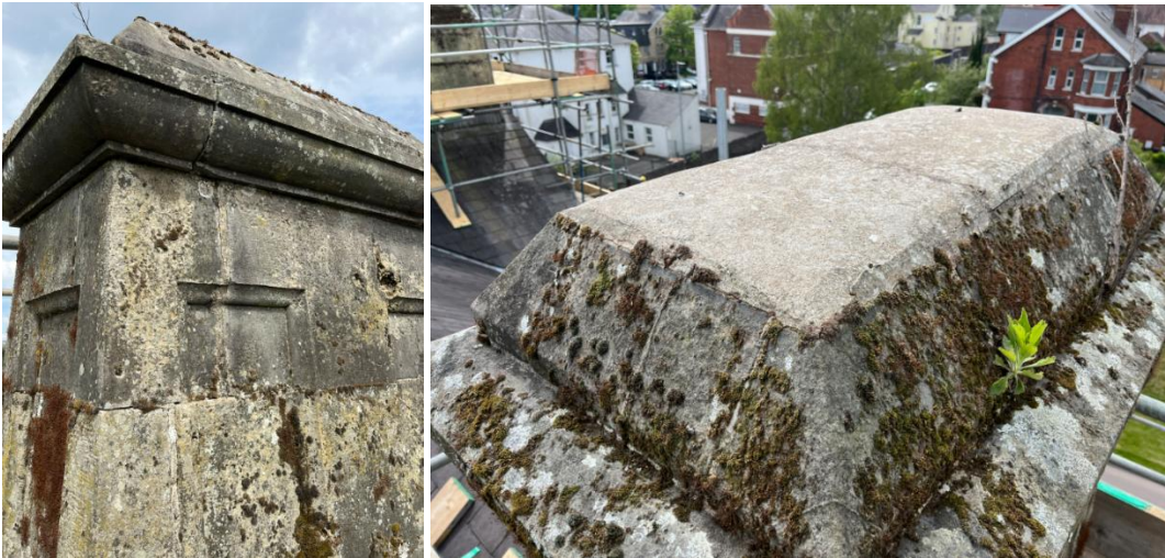
Plates 1-2: Close up pictures of PREVIOUSLY capped existing chimney, shows narrow cementitious flaunching on top of large slate (presumed).
