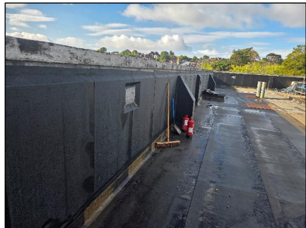
Figure 1-4 – Civic Centre Parapet
