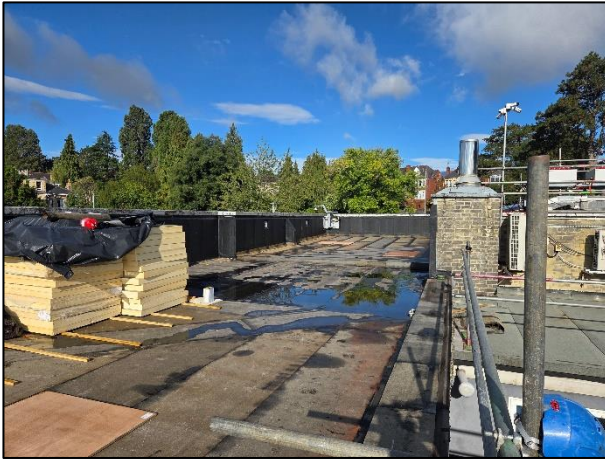
Figure 1-5 – Civic Centre Roof and Parapet
