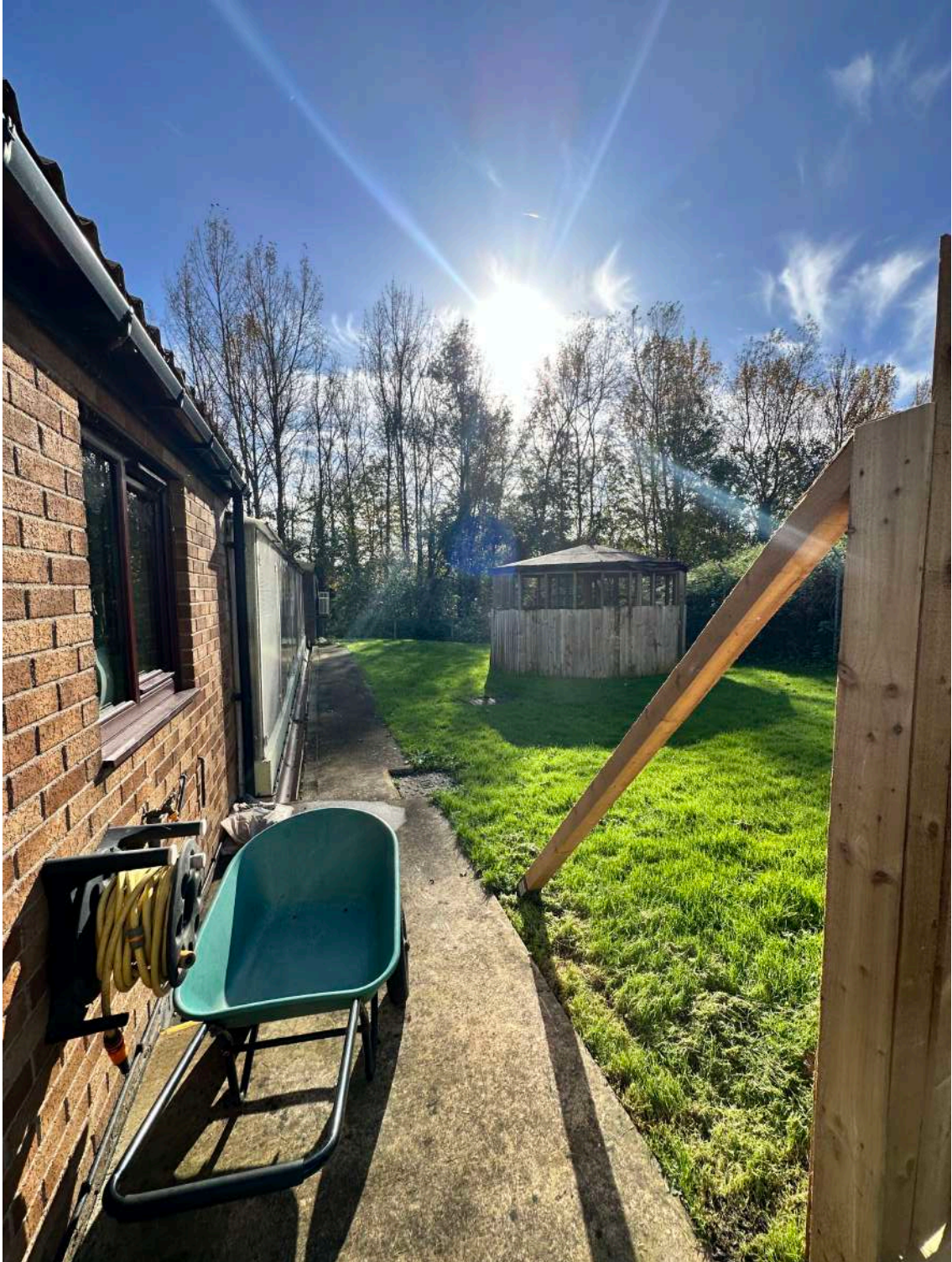
Photo E : View facing South with the external day spaces to the existing cattery isolation block on the left.
