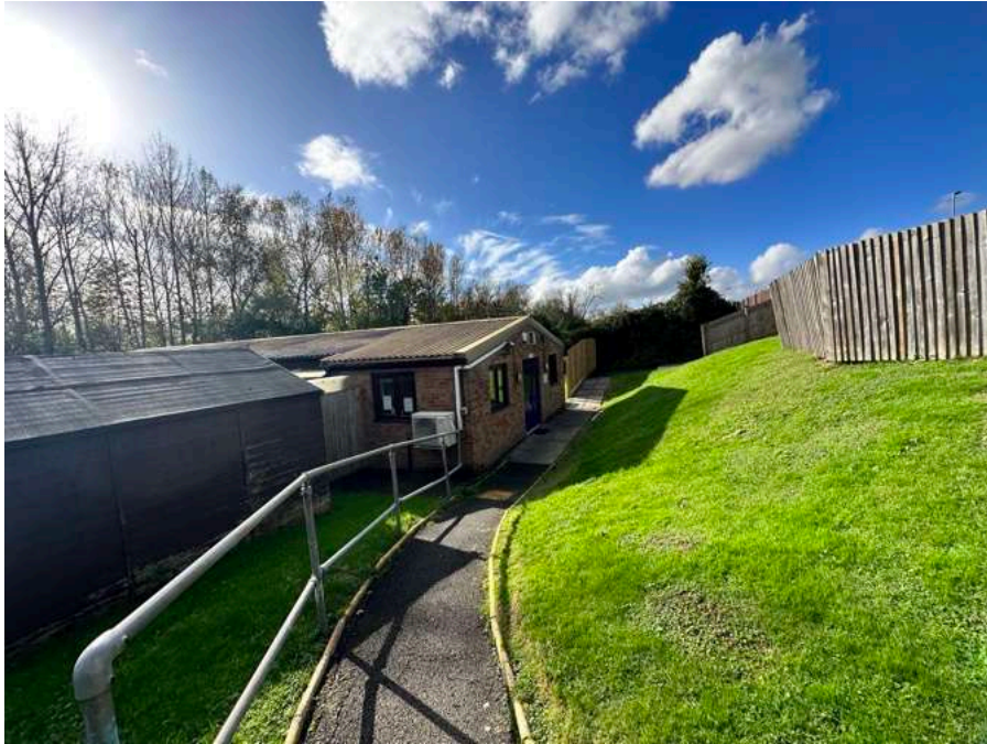
Photo C : Main entrance to the isolation cattery looking West
