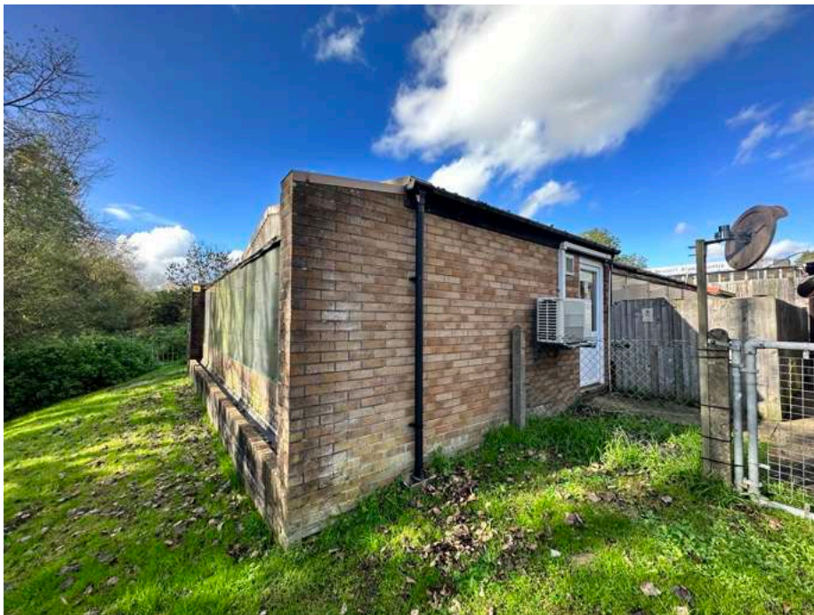
Photo G : View of the rear and side of the isolation cattery facing West.
