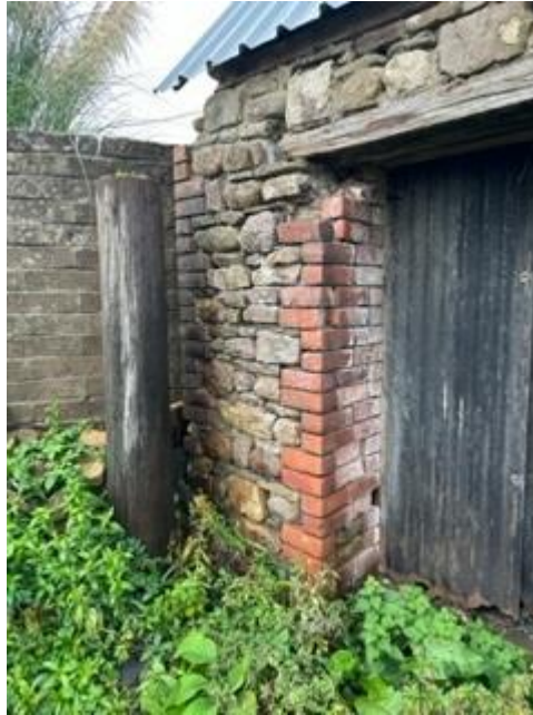
Figure 21 Brickwork reveals to structural opening.
