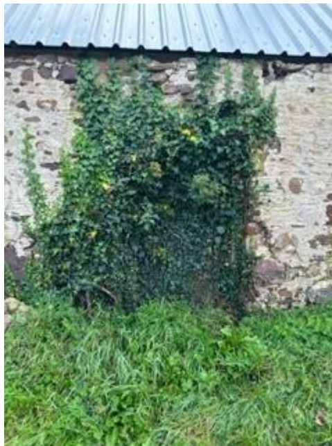
Figure 4 Front (Coc Y North Road) elevation 4 of 5
