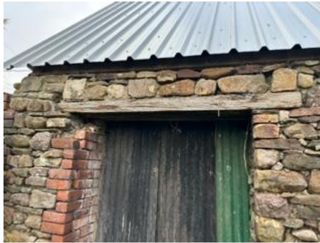
Figure 23 Lintel to structural opening.
