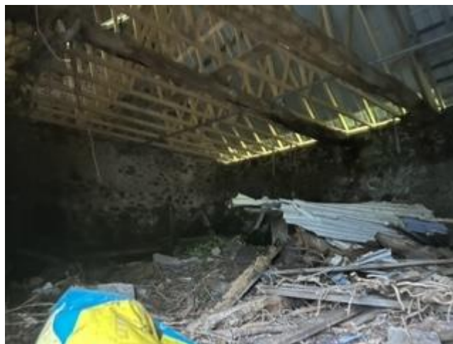
Figure 24 Trussed roof to right hand room.
