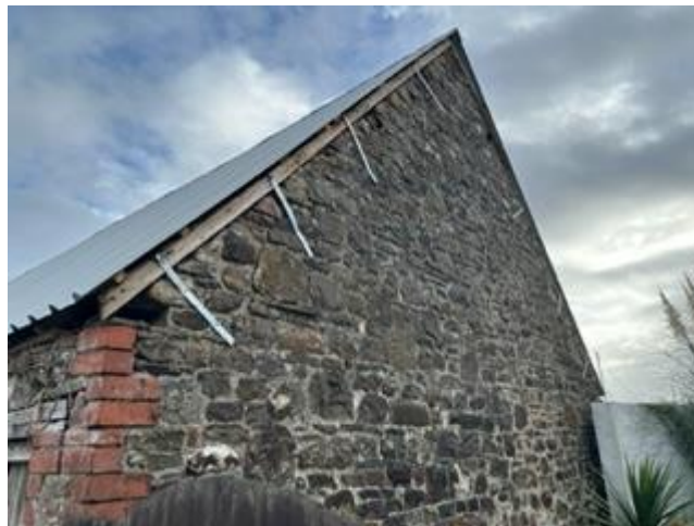
Figure 26 Right hand gable.
