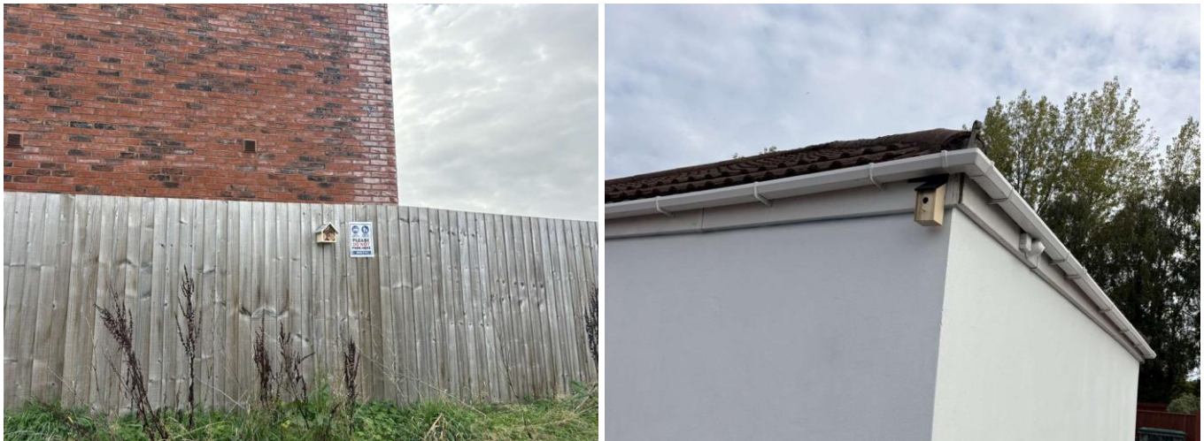
Images of erected bird nesting box and bee habitat box
