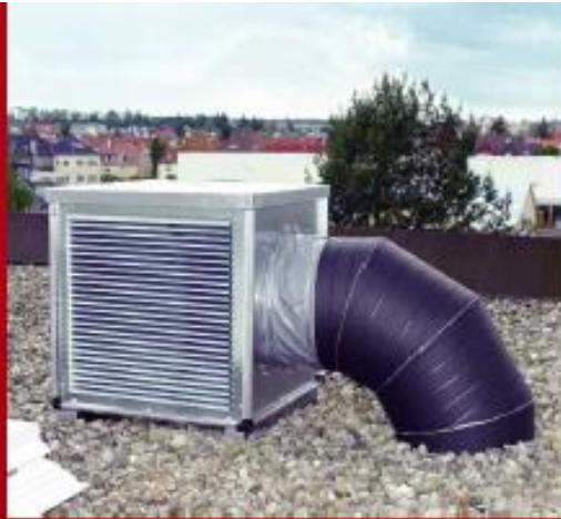
Roof installation with outdoor cover hood and external weather louvers (accessories).
