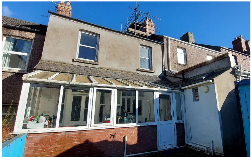
Figure 2 -Rear of property
