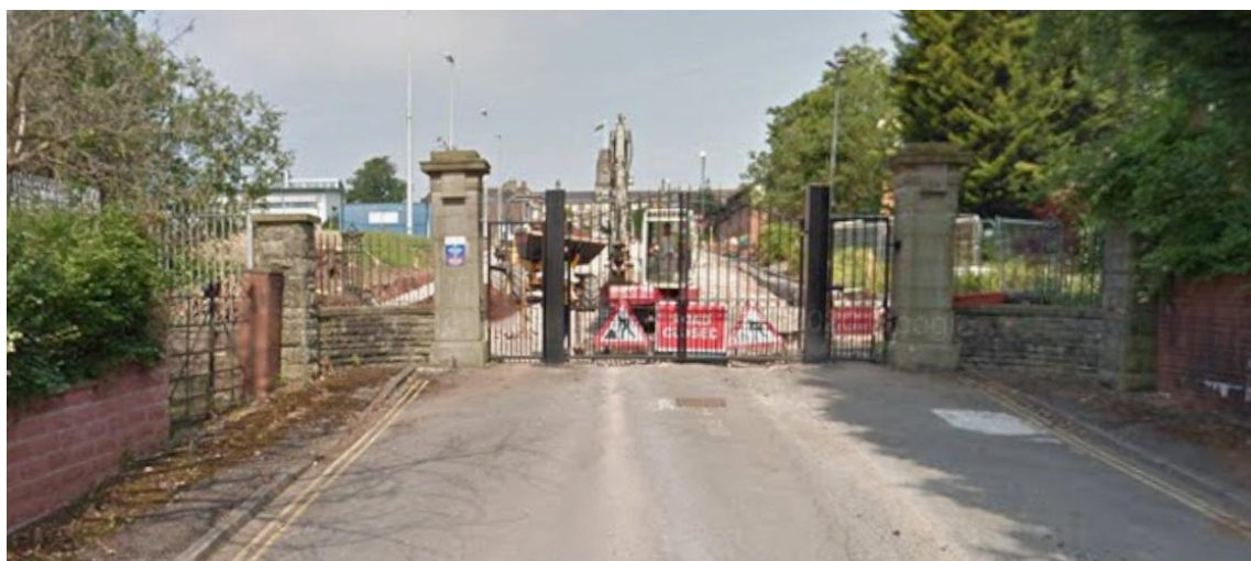
Figure 29. Replacement gates in 2012. (Google Streetview).
