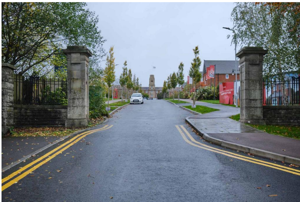
Figure 27. Gate piers at the entrance to College Road.
