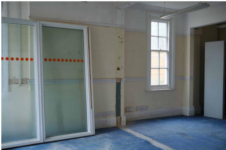
Figure 14. Interior showing position of a former fireplace.
