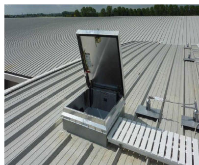
Roof access examples. (internal and external)
