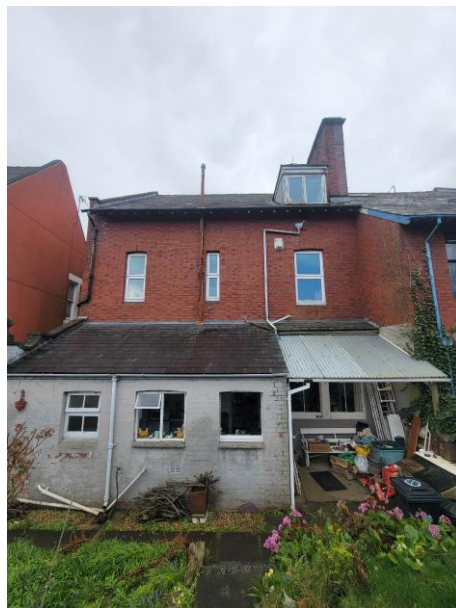
Fig. 6 – Rear Elevation of 31 Fields Road
