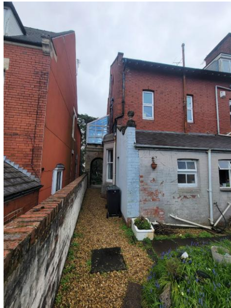
Fig. 5 – Rear Elevation of 31 Fields Road
