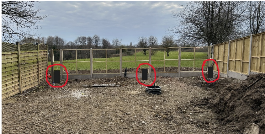
Photo of areas where 115mm core holes to be drilled for hedgehog run.
