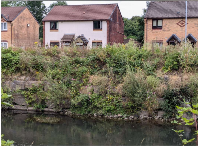
View of eastern bank from western bank, upstream of existing bridge
