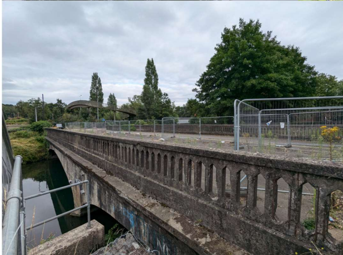
Existing bridge, view west to east over deck and upstream side
