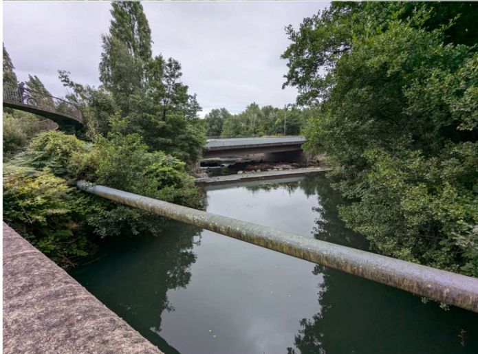
View downstream of existing bridge, from deck level, view over vegetation to be retained
