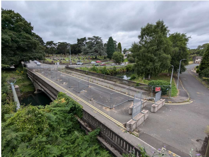
View towards north over existing bridge, from pedestrian walkway to east of structure
