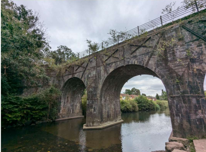
Offsite to north of viaduct, view to south-east
