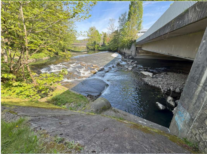
View upstream from western bank of A467 bridge
