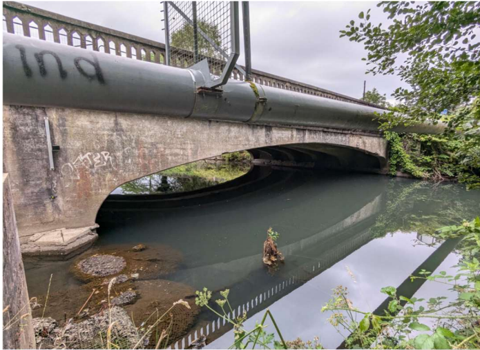
Downstream side of existing bridge, from western bank
