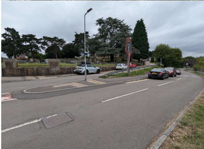
View towards churchyard and highway from western side of existing bridge
