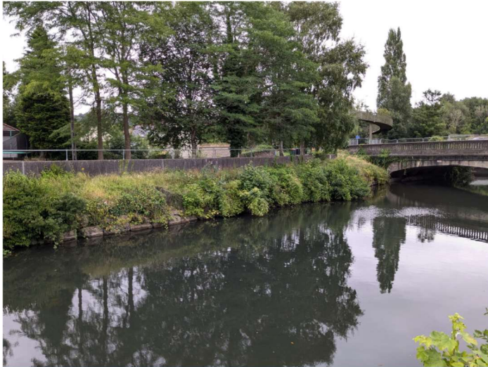
View of trees which will be removed, and upstream side of existing bridge from western bank.
