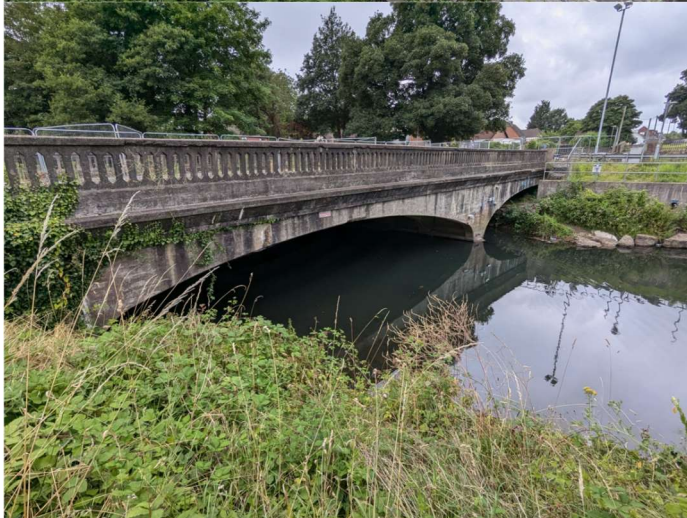
Upstream view of existing bridge from eastern bank
