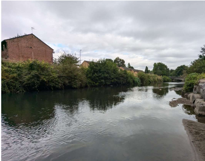
View downstream, from just downstream of viaduct
