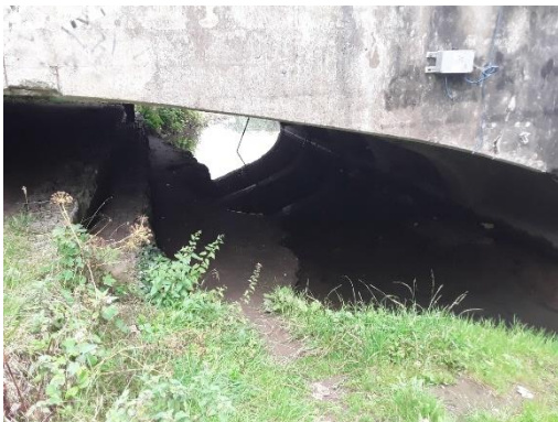
Figure A.21: View of gabion baskets beneath Bassaleg Bridge.
