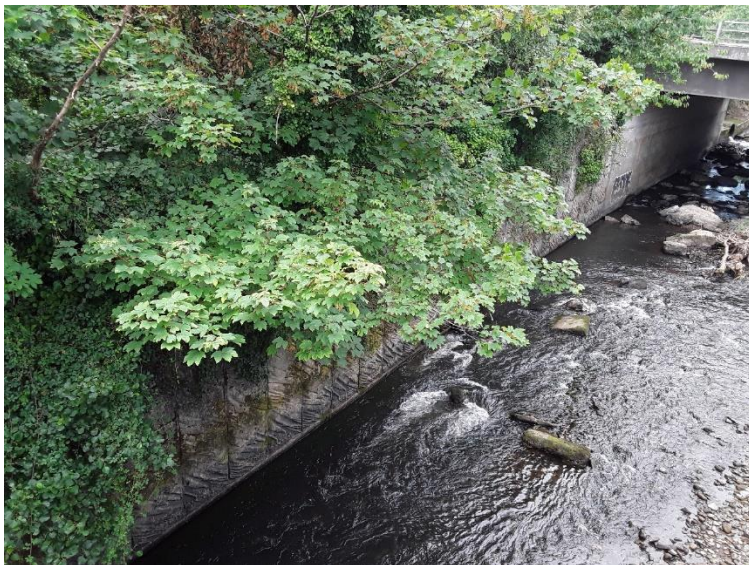
Figure A.25: View of Reach 3 concrete banks and substrate.
