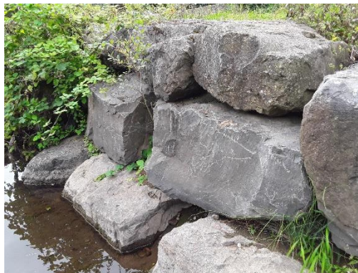
Figure A.22: View of blockstone reinforcing both banks
