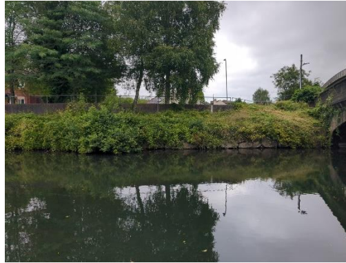
Figure A.14: Downstream facing view from upstream end of Reach 2.
