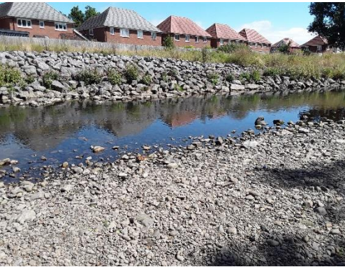
Figure A.41: View of rip-rap on left bank.
