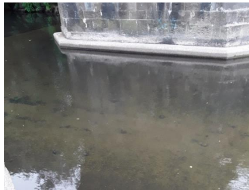
Figure A.12: View of concreted river bed below railway bridge.
