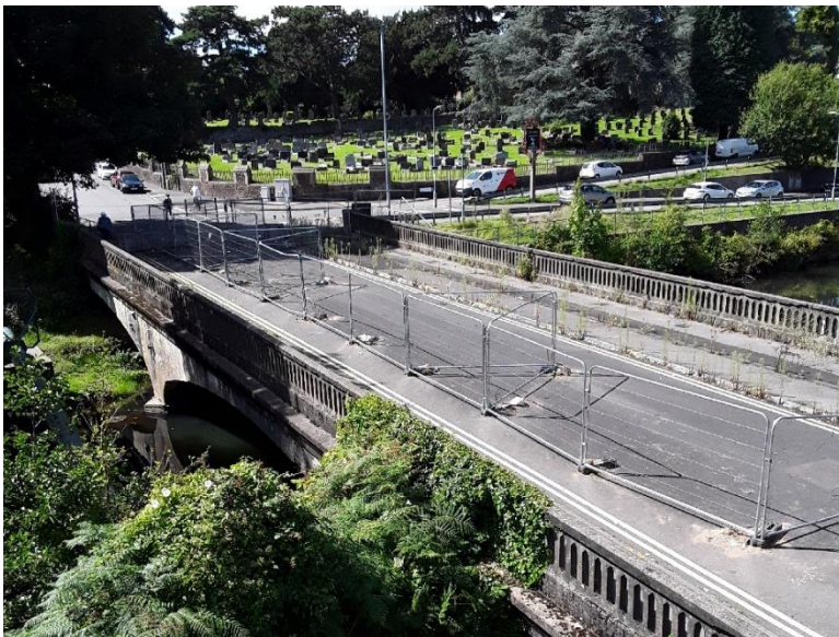
Figure 1.1: Image of the old Bassaleg Bridge.
