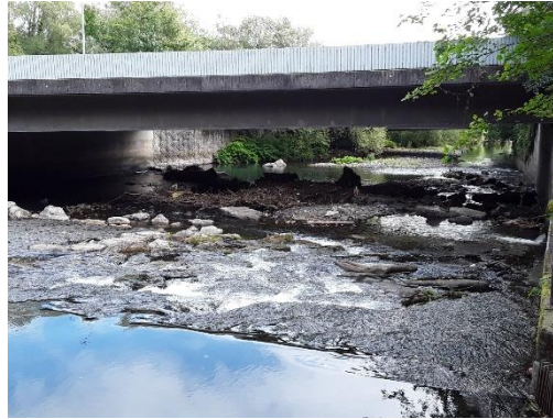
Figure A.24: Downstream facing view from upstream end of Reach 3.
