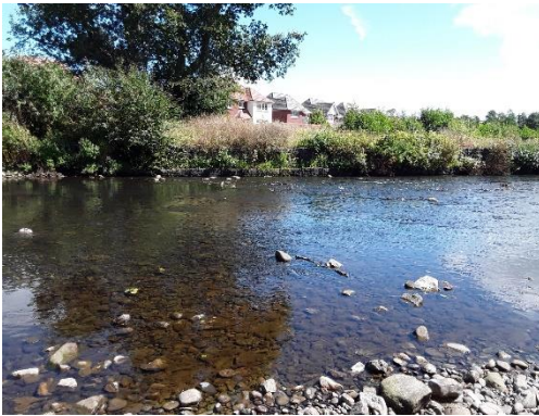
Figure A.40: View of gabion baskets further downstream on left bank.
