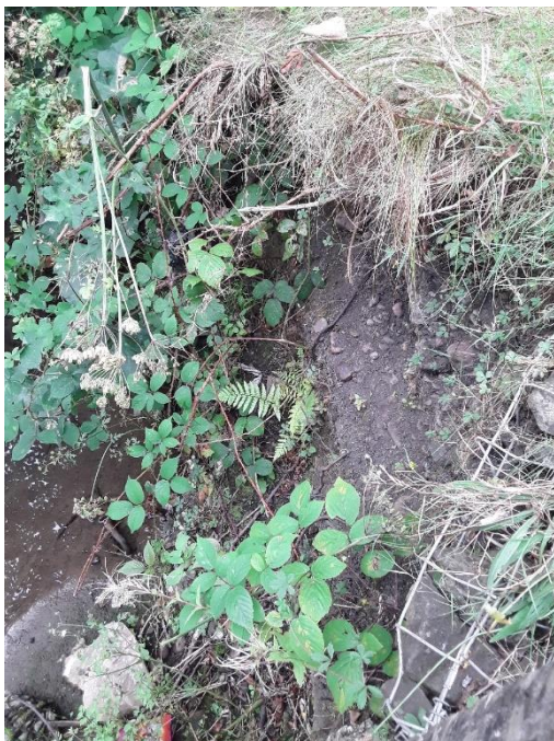
Figure A.15: View of Reach 2 bank materials near eroded area.
