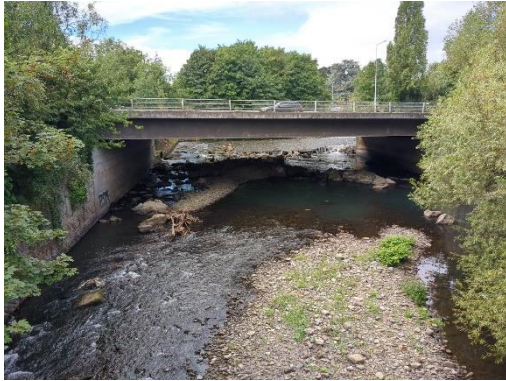
Figure A.26: Upstream view showing both mid-channel bars.
