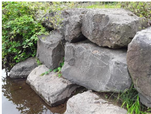
Figure A.22: View of blockstone reinforcing both banks
