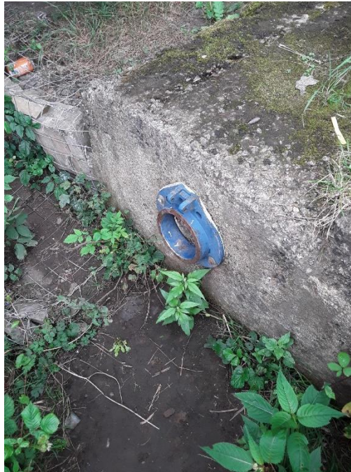
Figure A.20: View of drainage outfall.
