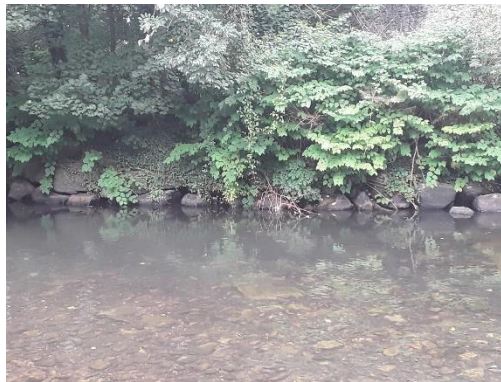
Figure A.18: View of left bank vegetation, including Japanese Knotweed.
