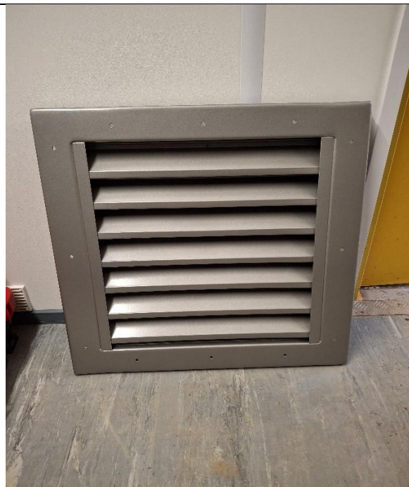
Fig. No.2b: Front of Intake 1& 2 damper Louvre (horizontally mounted blades)
