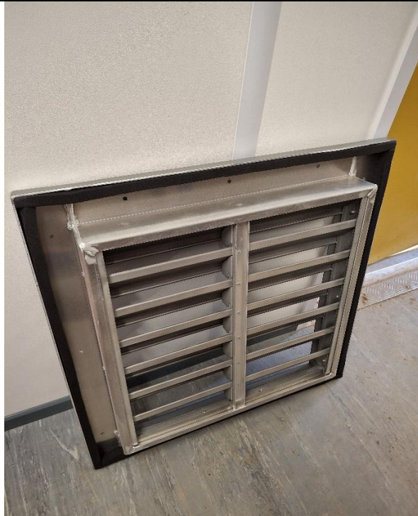
Fig. No.2a: Rear of Intake 1& 2 damper Louvre (horizontally mounted blades)
