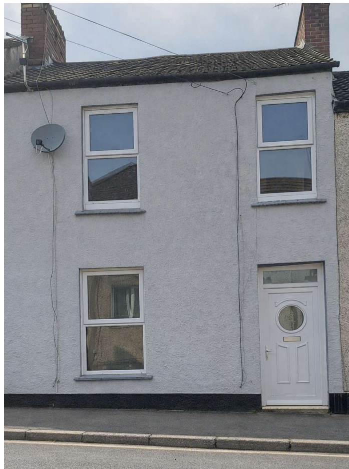
Photo 1 – Front of property
