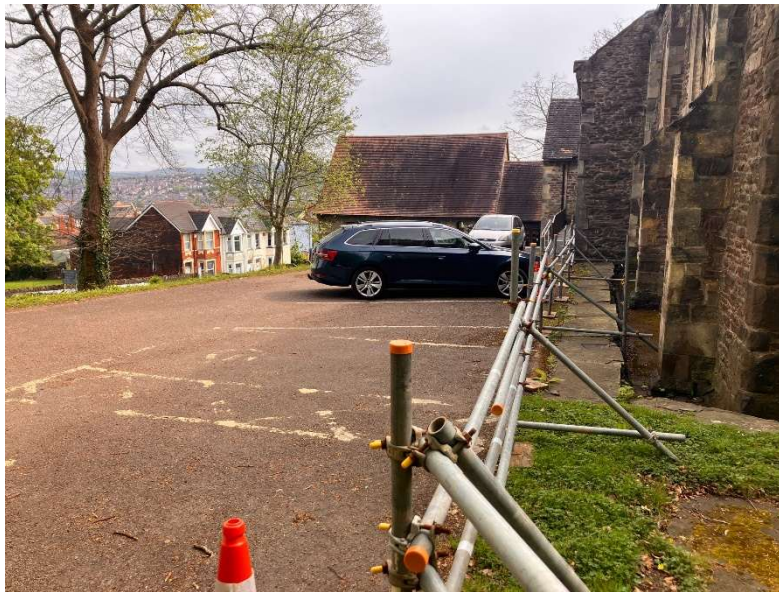
Parking area separated from the North Aisle by sunken drainage channel, edged with ledger stones. Note the temporary fall protection currently in place.
