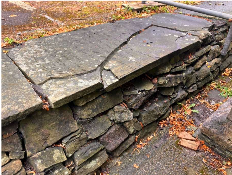
Condition of ledger stone on north side of North Aisle.
