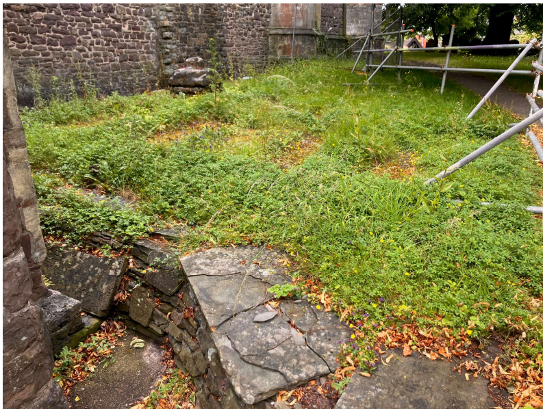
Grass area in front of the Galilee Chapel, which is to be retained as existing, i.e., with no guarding to the drainage channel and ledgers retained in-situ.
