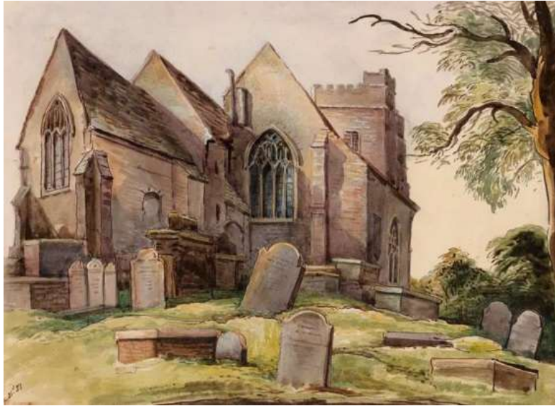
Painting, dated 1853: NE area of churchyard showing many burials, all of which was removed during building of Vestry buildings and Chancel in the 20 th Century.
