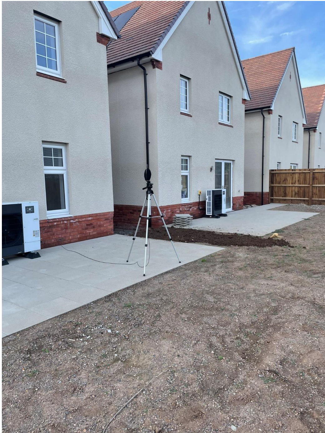
Figure 2 – View of Equipment External Location Plot 9
