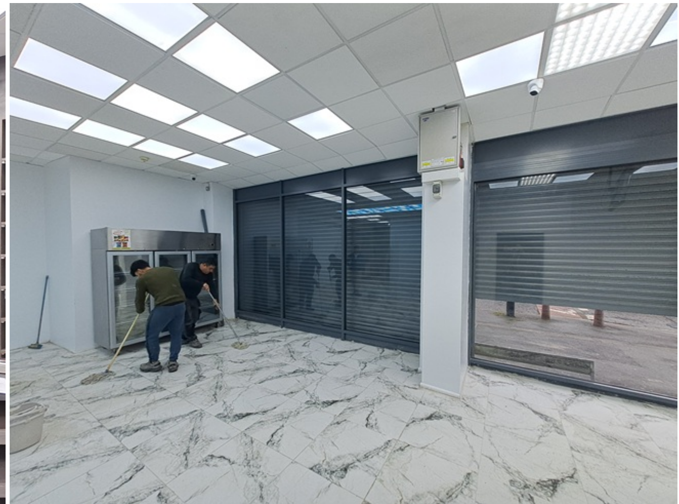
Photo 4 – New Flooring and shop front
