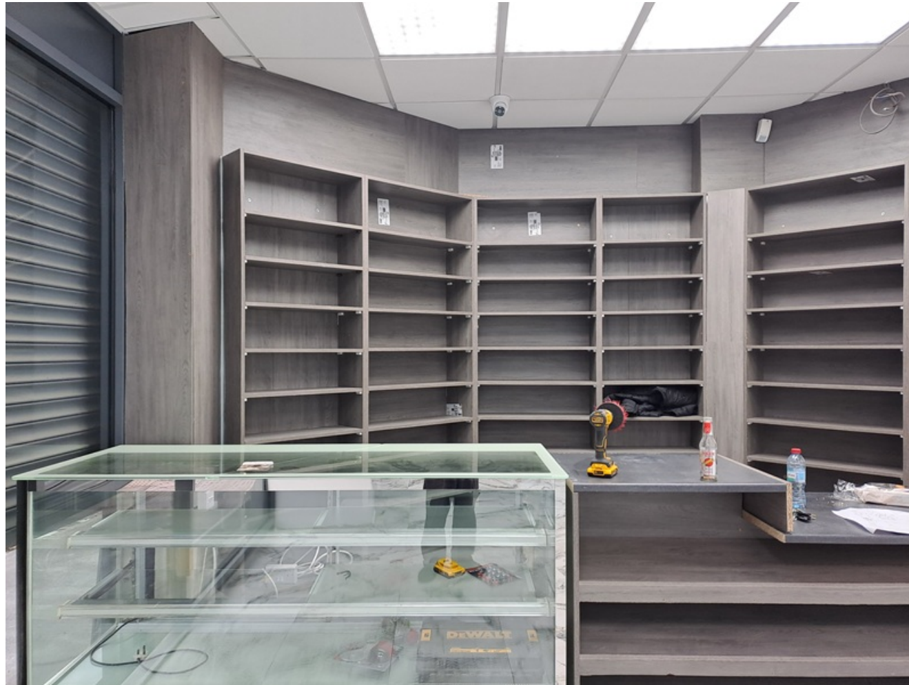
Photo 3 – Shop Fit out
