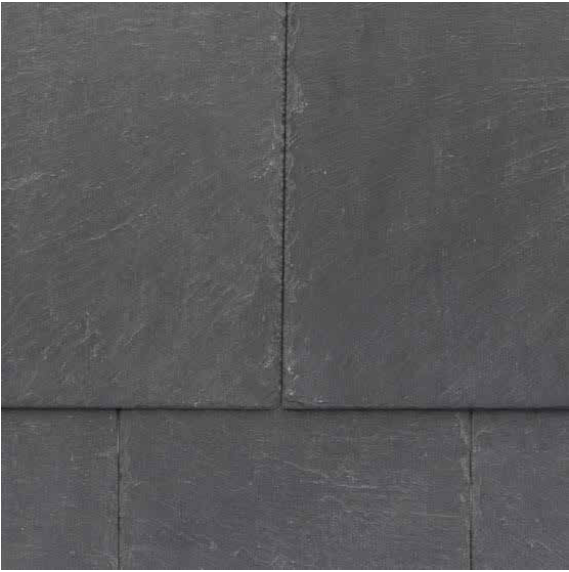
Block A Pitched Roof Pizarra's Cupa12 Natural Slate
