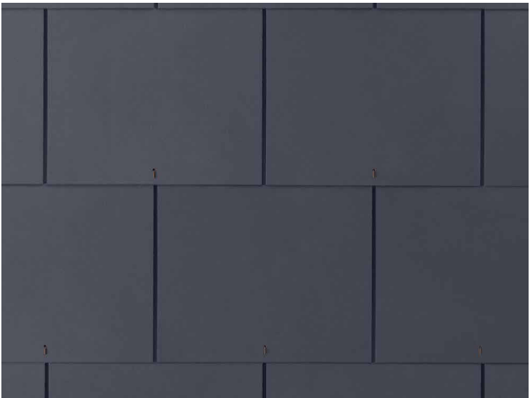
Block B Pitched Roof Blue/black colour Thrutone fibre cement roof slates
