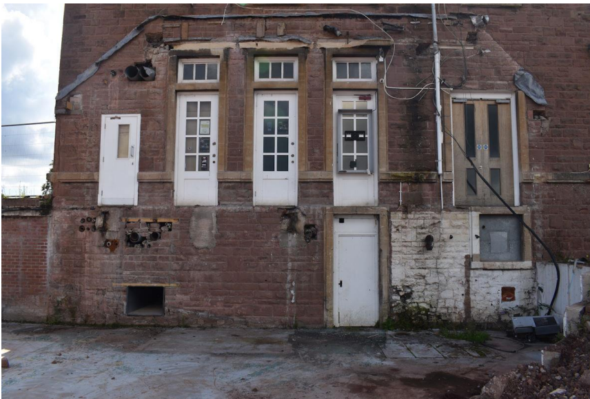
Figure 4.1: Northeast elevation of the main teaching college following removal of extension.
