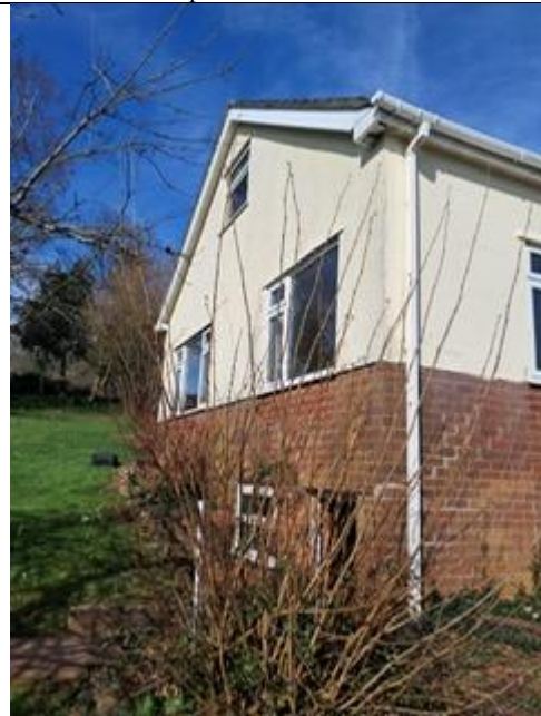
Photo 9: West face of house with undercroft
