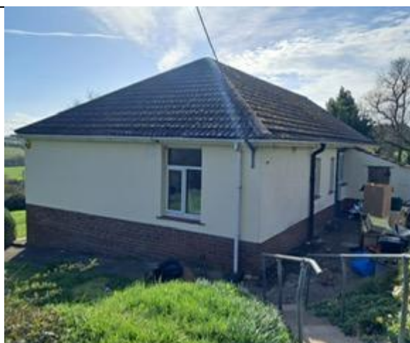
Photo 16: East side of house
