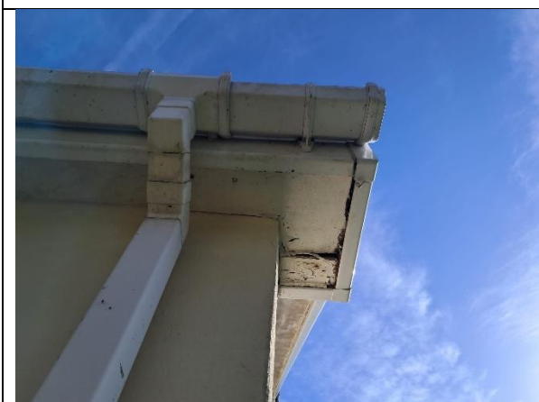
Photo 13: west facing soffits
