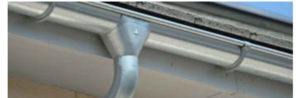
Material: GALVANISED STEEL Colour: SILVER Location: RAINWATER GOODS
