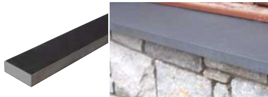
Material: SLATE/SANDSTONE Colour: GREY Location: LEDGE BETWEEN STONE + RENDER ABOVE
