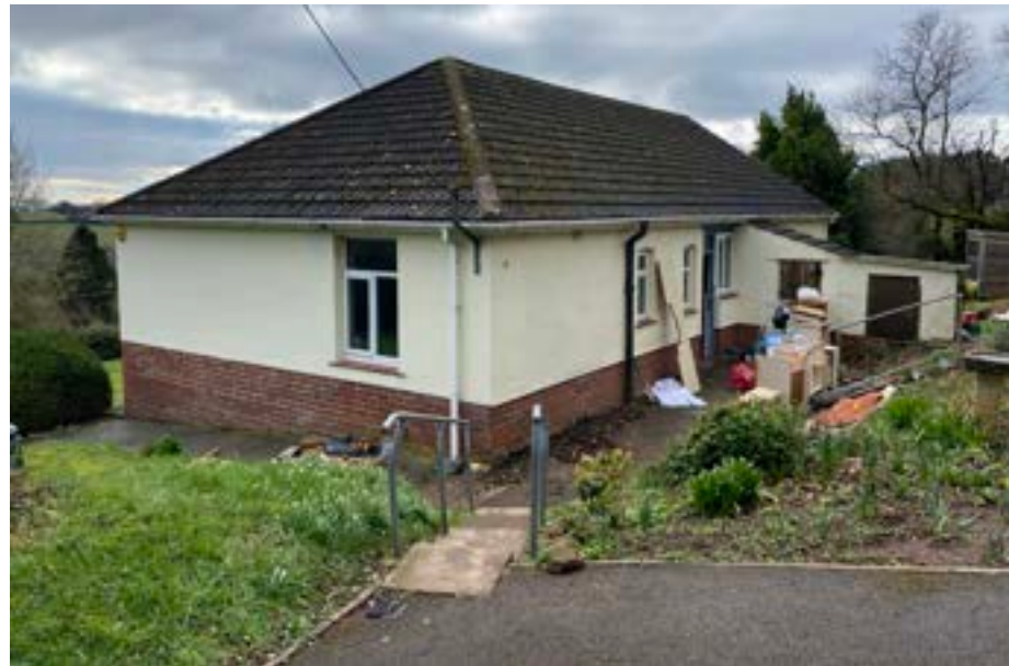
Existing bungalow - approach from above - north east corner
