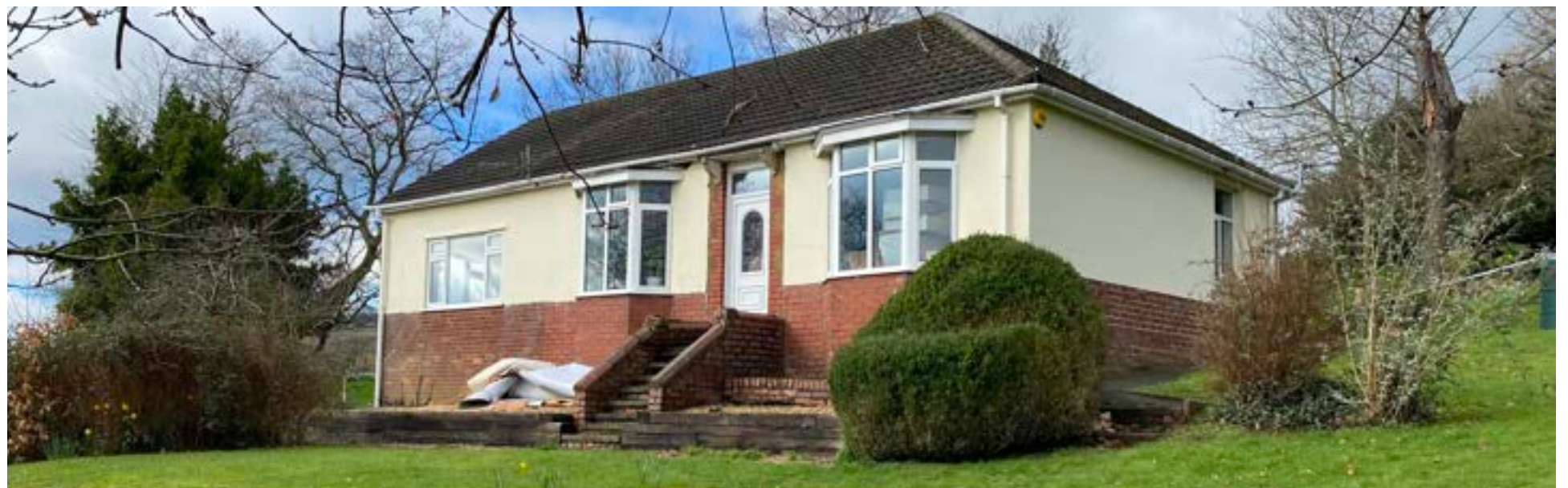
Existing bungalow - approach from below - south elevation
