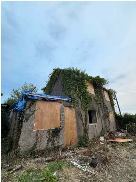
Plate 2 Surveyor View, Southern Gable
