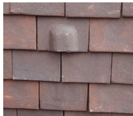
Fig 1 – Example of Bat Access Tile
