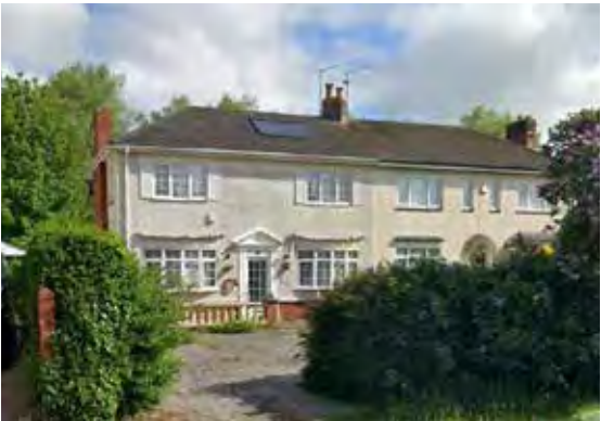
Solar Panels Visible
