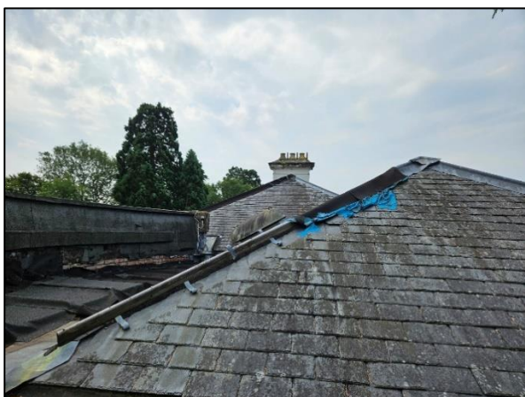
Figure 4-11 - Roof Hip Repair
