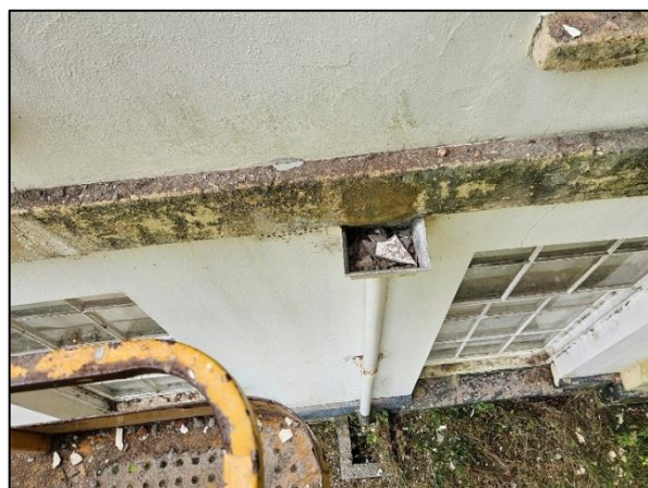
Figure 4-6 - Blocked Gutters
