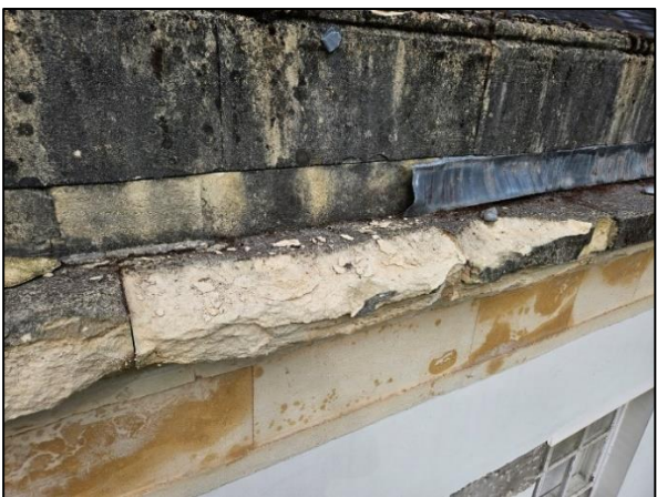
Figure 4-5 - Weathered Coping Stones
