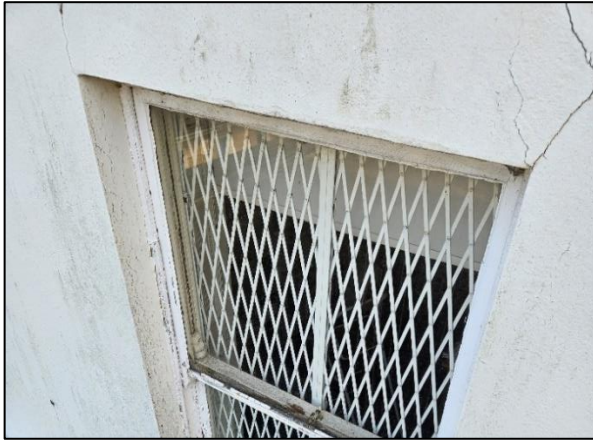
Figure 4-1 – Window Cracking
