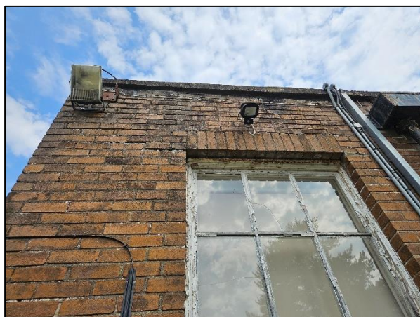
Figure 4-17 - Soldier Overhangs Steel Lintels
